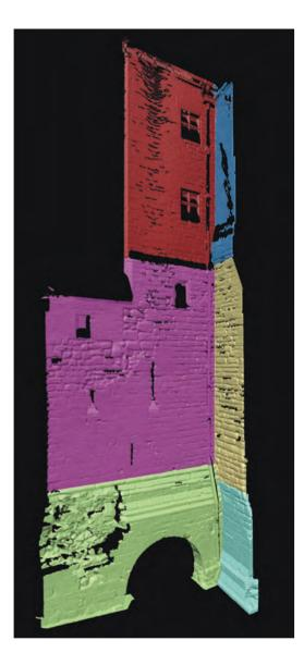
Fig 1.5 Laser scan survey of the Black Gate, 2009 (collaboration with the University of Northumbria, School of the Built Environment).
