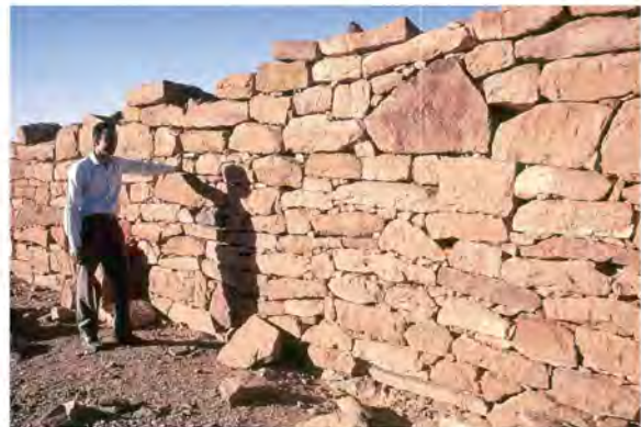
Figure 1.7. The outer (western) face of wall ZIN900.001, showing the close jointing and the centrally placed large polygonal block in distinctively dark stone (a decorative feature?) (CMD 1973).
