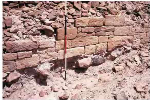
Figure 1.76. Detail of ashlar footings of wall ZIN003.007, looking north (CMD 1965).
