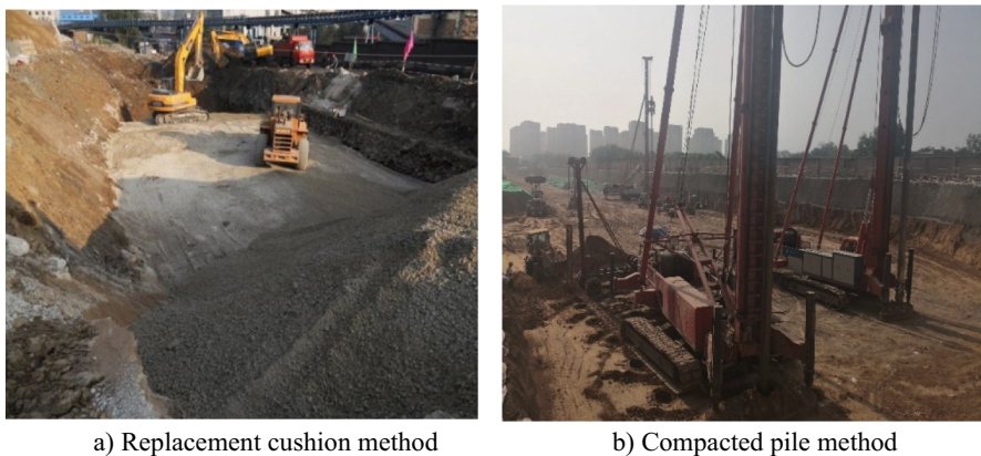
Fig. 2. Some foundation treatment methods
