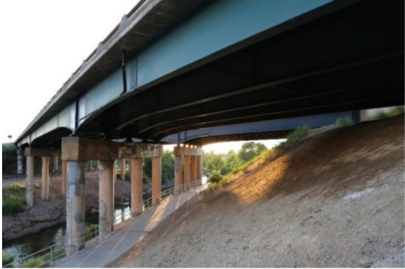
Fig. 1. Bridge examined in this study.
