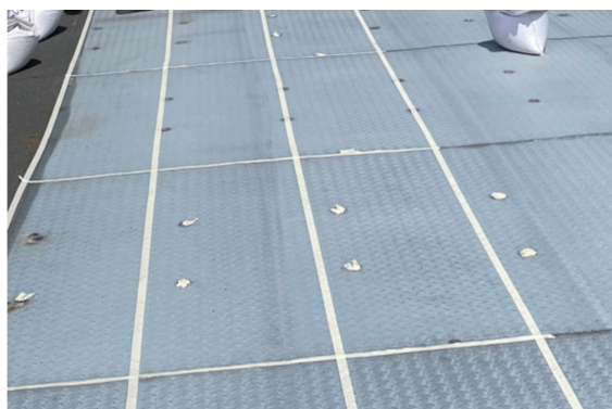
Fig. 6. Treatment of seam leaving at anchor bolt
