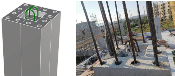
Fig. 7. Bellows through hole prefabricated column
