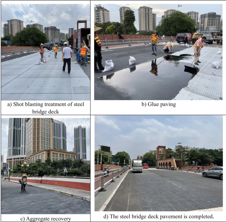
Fig. 7. Steel deck pavement of bascule bridge
