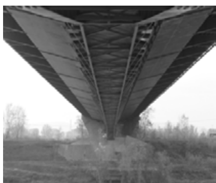
Figure 10.9 Sight of the bridge from below.
