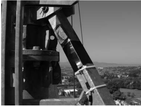
Figure 7.3 Strain gauge on the diagonal element of the truss system protected from the environmental conditions..
