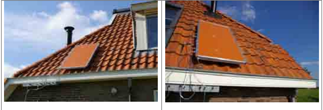
Figure 2 (left) Panel 1, located on southern roof pitch; Figure 3 (right) Panel 2, located on western roof pitch. The gray boxes under the gutter contain the pressure transducers. Pressure taps are present at the vertical centre line, at \frac{1}{4} , \frac{1}{2} and \frac{3}{4} of the height of the panel, both on top and on the bottom.
