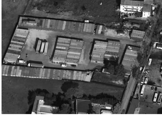
Fig. 7 - Containers used as storehouses
