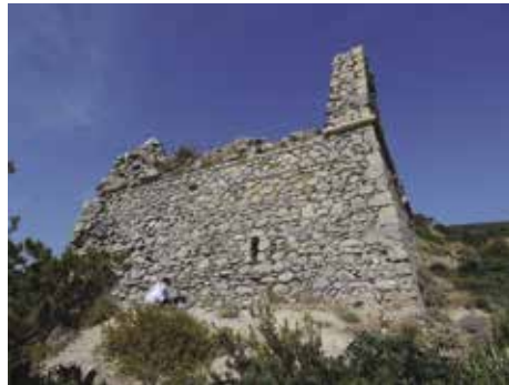
Figure 6 – Tower of Calamoresca, Argentario.
