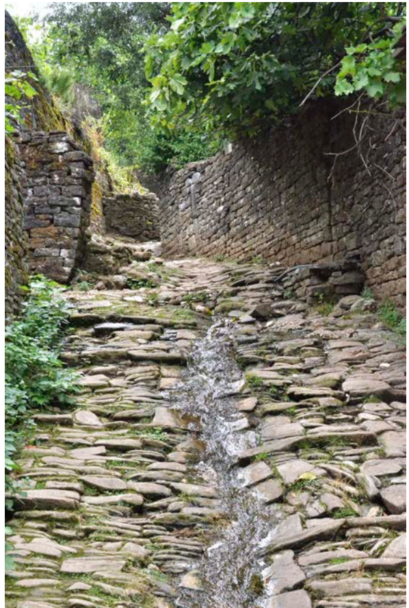
Figure I-4.3.1 – The main street of the village paved in kalldrëm and its water drainage channel in the middle.
