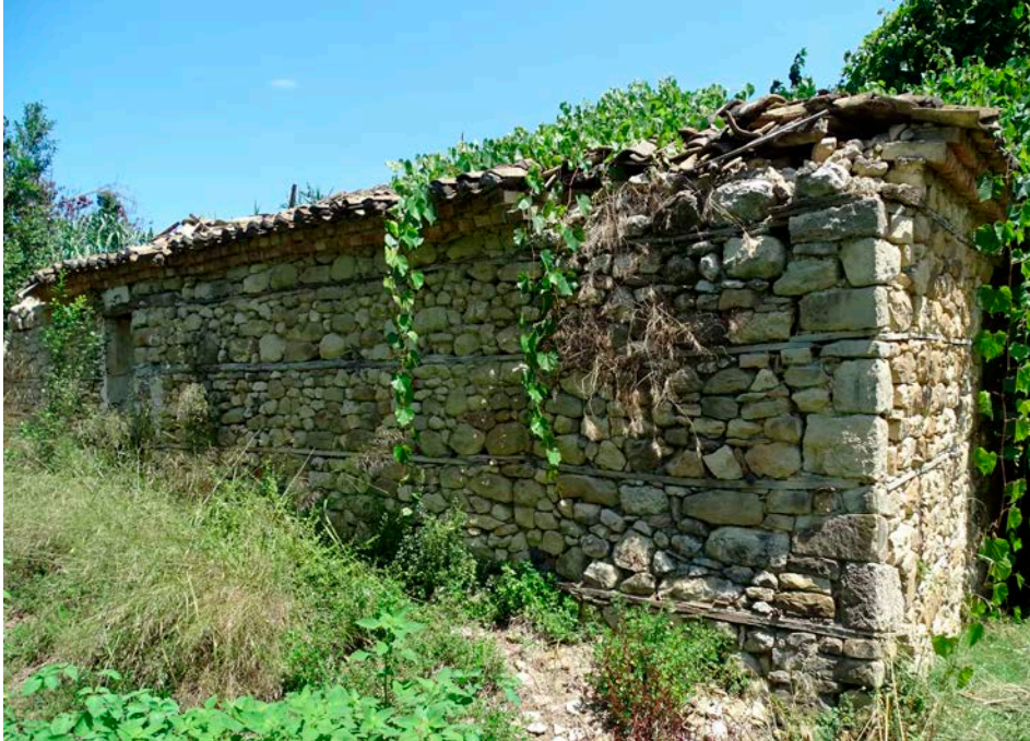
Figure III-4.2 Remains of a traditional dwelling in the hill quarter with horizontal reinforcing timber elements.
