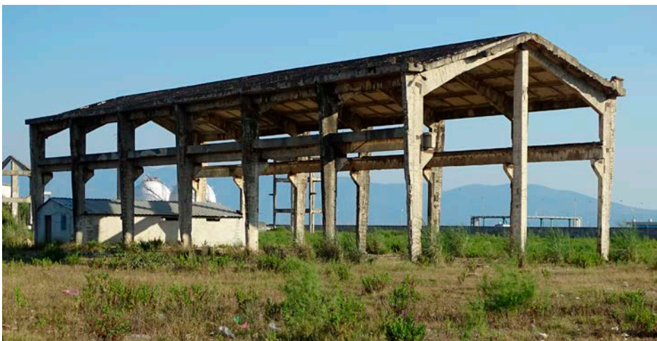
Figure III-3.8 – Above and on the next page: Remains of the former Uzina PVC plant.
