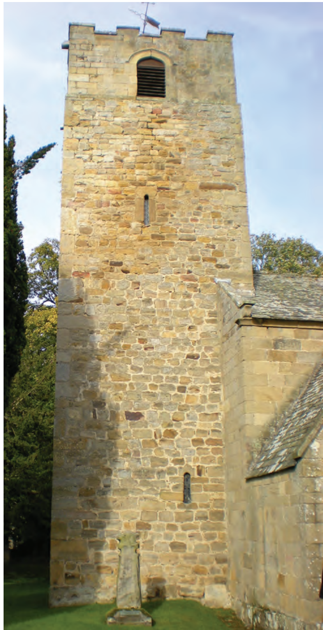
Figure 9.16. The tower at Warden church, Tynedale, probably constructed during the seventh century in stone, of which some has evidently come from Hadrian's Wall which lies just 4km distant. Note the Anglo-Saxon cross-shaft in the foreground.
