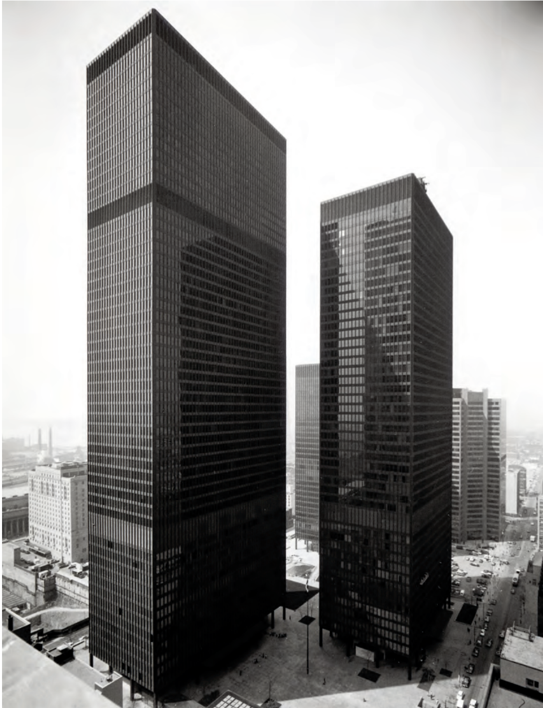
6.20. Toronto-Dominion Centre, Toronto, Panda Associates fonds, Canadian Architectural Archives (PAN 74236-4C).
