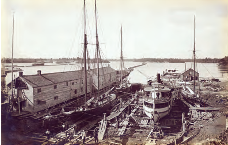
Fig. 2.10. Muir Bros Drydock Company, 1882. (Photo: Brock University Special Collections and Archives.)
