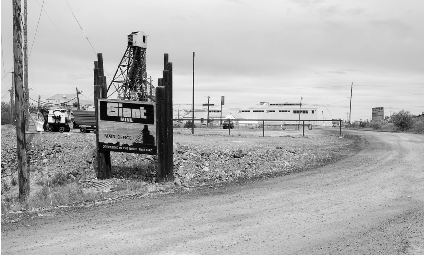
FIGURE 2: Yellowknife, NWT's abandoned Giant Mine in 2008, before remediation activities began. Remediation costs at Giant are expected to exceed $1 billion. Photo by Arn Keeling.
