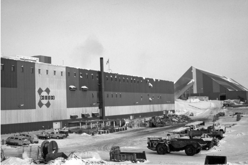
FIGURE 3: The Polaris Mine. NWT Archives/Northwest Territories Dept. of Public Works and Services fonds/G-1995-001: 1525
