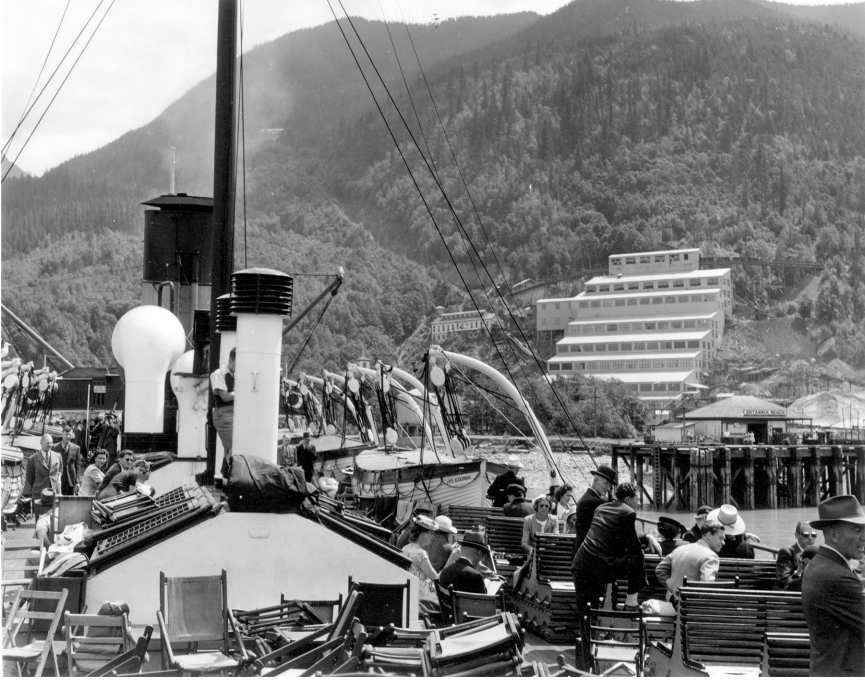
FIGURE 8.5. Excursionists aboard the Lady Alexandra . As shown, they are not paying much attention to the Britannia Mine, which was advertised as a feature attraction on the tour of Howe Sound. Courtesy of City of Vancouver Archives.
