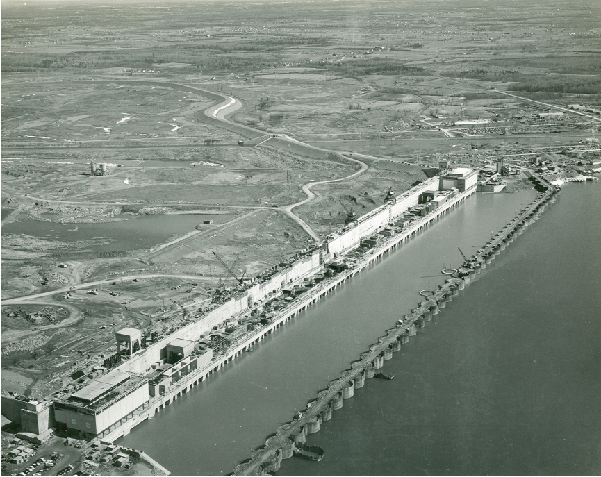
FIGURE 5.2. Moses-Saunders dam under construction, c. 1956. Courtesy of Ontario Power Generation.
