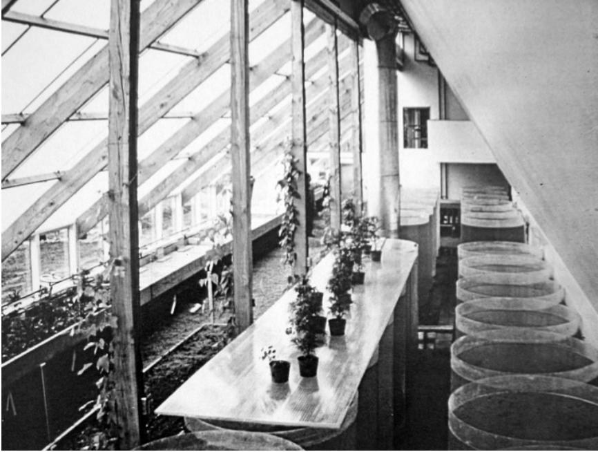
7.4 The PEI Ark's greenhouse. The large plastic cylinders are solar algae ponds for raising fish and moderating the greenhouse temperature. Source: An ARK for Prince Edward Island .
