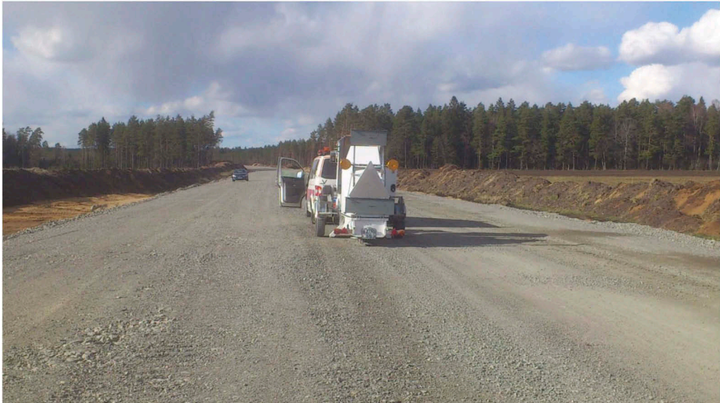
Figure 1. Testing on the subbase in April 2012.
