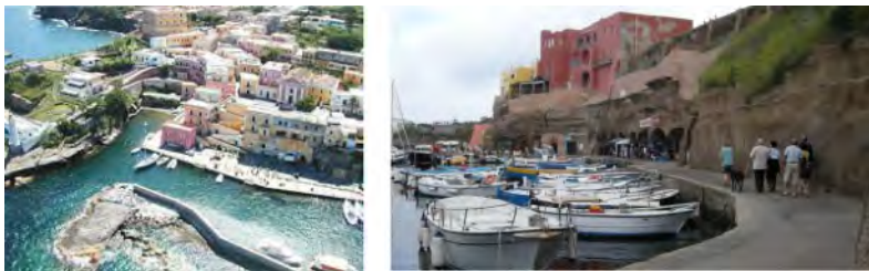
Figure 7. The Roman port of Ventotene (one of the Pontine islands, Italy), still in use (thus at the highest possible level of functional integrity), was entirely excavated in the rock bank, removing some 60.000 m 3 of material, to support emperor Augustus' (63 BC – AD 14) summer residence, as there was no natural harbour on the island.
