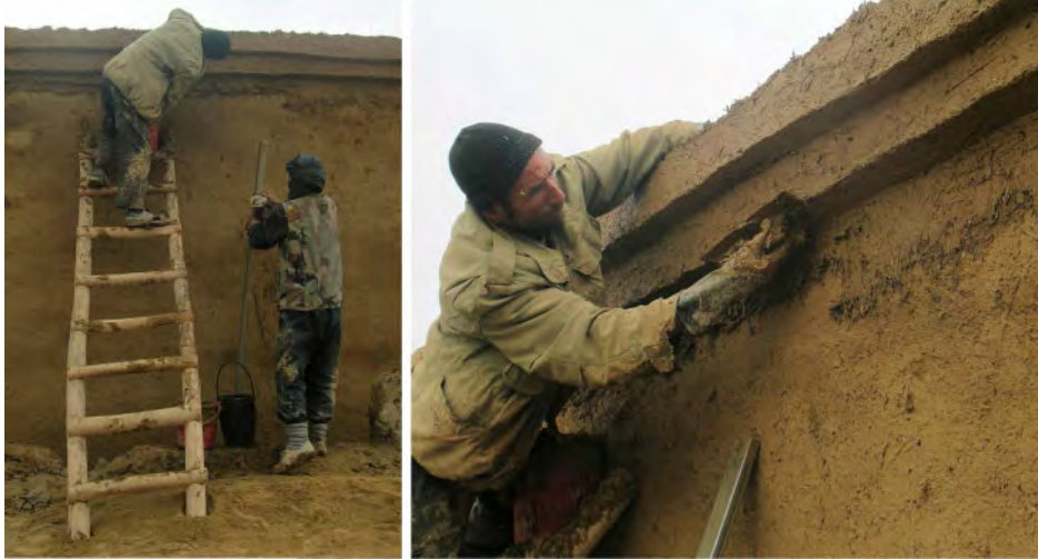
Figure 8. Wall repair. Bamiyan, Afghanistan. Ph.: P. Smars, 2003.
