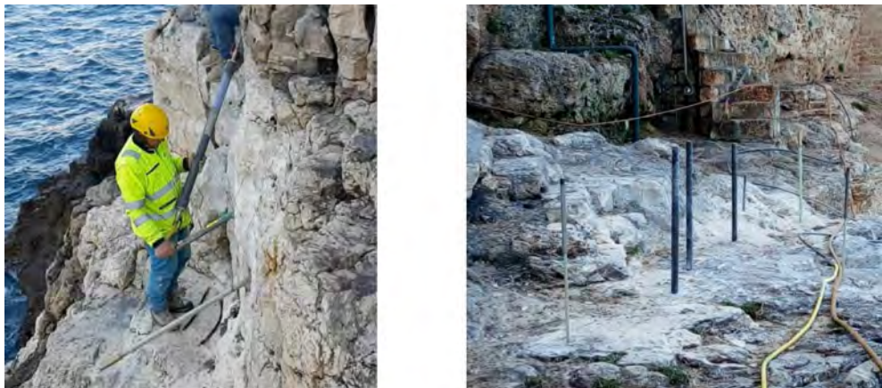
Figure 9. a) Technician during injection MasterEmaco A 60 in CB1/2; b) anchor in FT2 zone 1.
