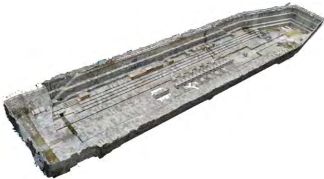
Figure 7. Perspective view of the 3-D texture model viewed from southern direction. The size of the dock, the length 134 m, the width 30 m, and depth is about 9 m.
