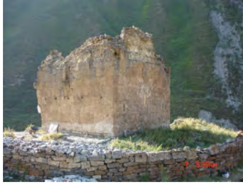
Figure 4. View of the church from South-East.
