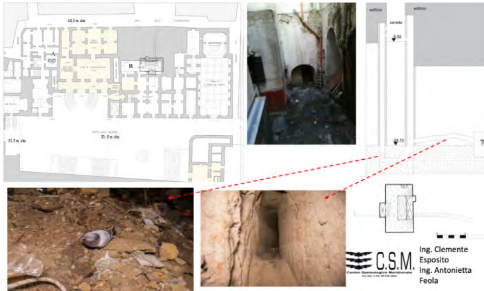
Figure 17. Shafts, cavities close to the Incurabili Pharmacy foundations.
