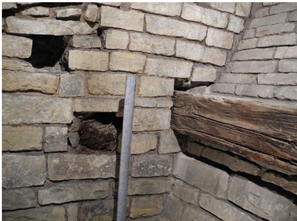
Figure 11. The wooden ties intersect at the corners of the octagonal plan of the Baptistery; the image shows the change in material of the dome at the level of the tie: below the masonry is stone, and above brick.
