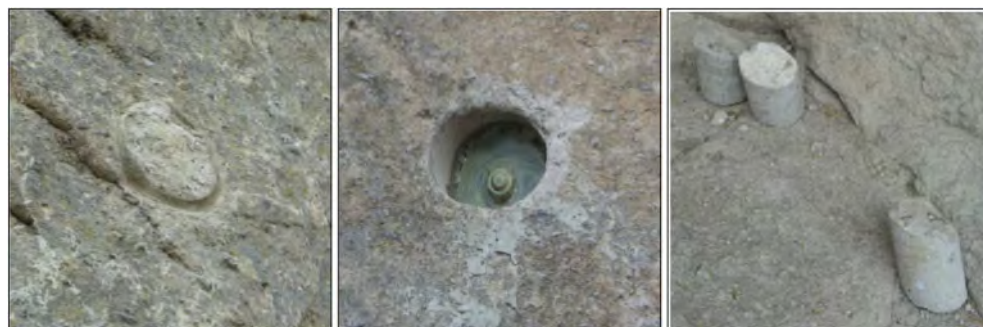
Figure 8. Rock core drilled used for mitigation (left), bar insertion (center) and bolt sealing (right).
