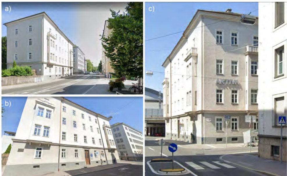
Figure 4. Overview of the building in Salzburg: a) north side of the building; b) west side and main entrance of the building; c) south side of the building.
