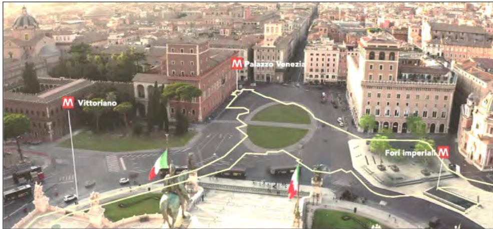
Figure 1. A view of Piazza Venezia with the projection of the Venezia stations.
