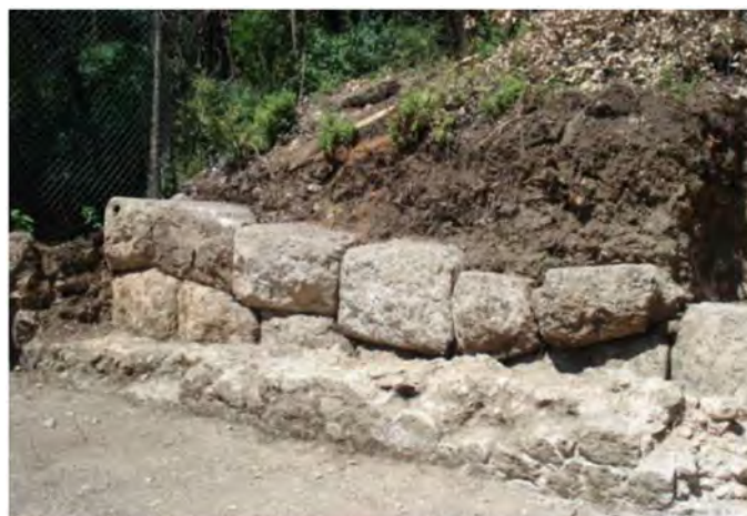
Figure 6. Picture of the polygonal wall (c). The geometrical model implemented in the analysis evolves as described in Figure 7 (from b to e).
