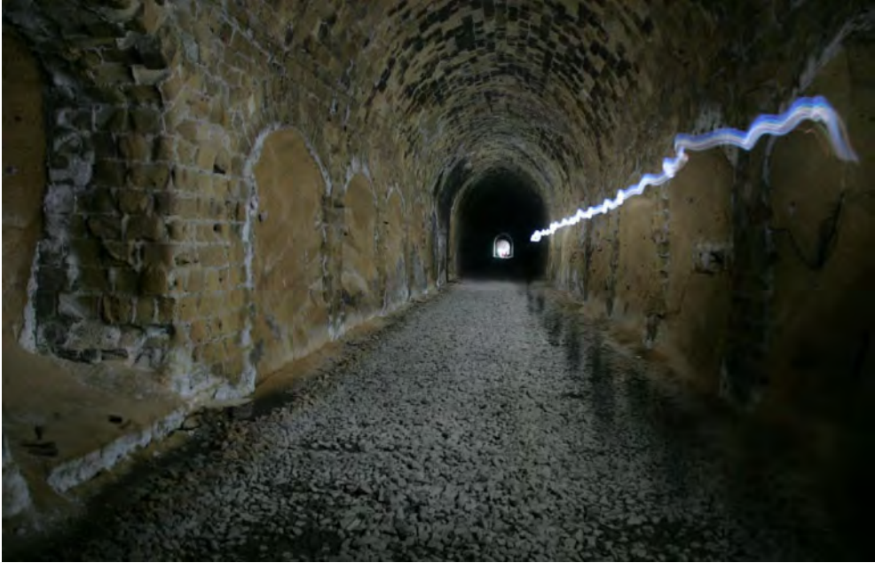
Figure 3. The dismissed Punta Epitaffio tunnel with the tuff layers exposed (photo by M. Fagnola – Cocceius Association).
