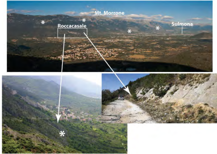
Figure 2. Panoramic view of the Sulmona Plain. Asterisks indicate some places where Mt. Morrone fault is emerging. Rectangle defines the area of Mt. Morrone bedrock fault scarp north of Roccacasale and the place where the fault plane is exposed south of the village.
