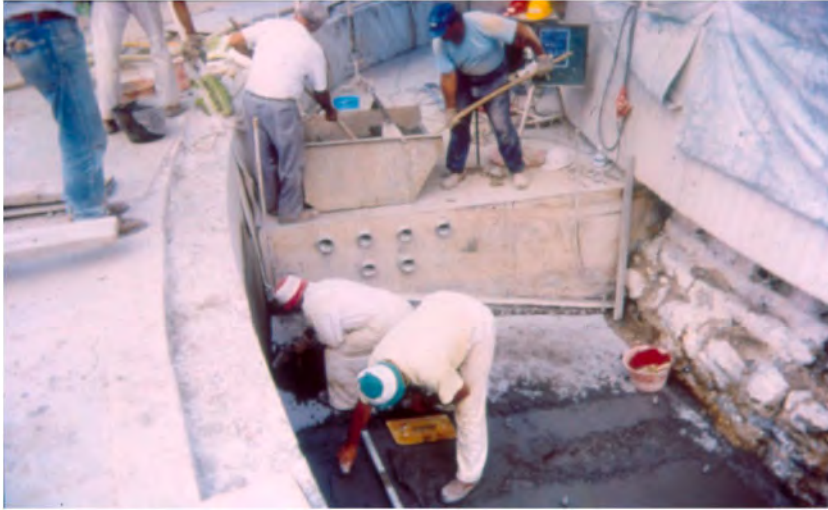
Figure 9. Construction of the northern sections of the ring beam for the ten anchors.
