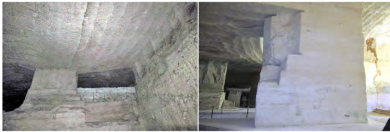
Figure 3. Western tunnels: bands, fan-shaped, and herringbone traces.
