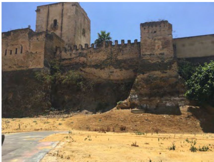
Figure 5. Sandblasting of the surface of the Utrera Castle.
