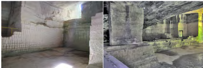
Figure 4. Eastern tunnels: cross traces in the lower part and traditional tools traces in the upper part.
