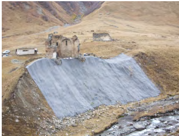
Figure 6. View of the church after the first part of emergency works.
