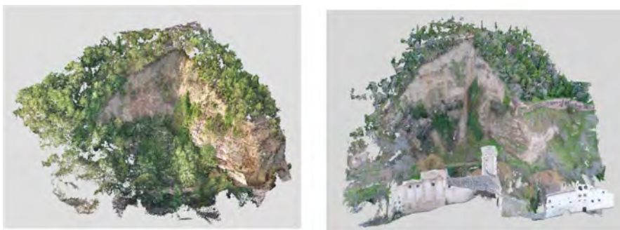
Figure 6. UAV photogrammetry monitoring results in the San Pedro cliff. Dense point clouds. Left: July 2017. Right: February 2018.
