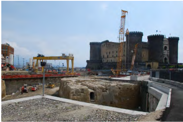
Figure 14. Excavation for a Metro station in Town Hall Square.
