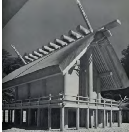
Figure 2. Ise shrine (Japan), which still undergoes ritual reconstruction every 20 years ever since the 7th century.
