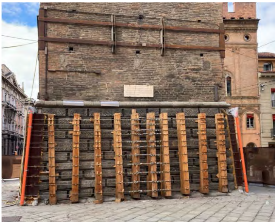
Figure 6. Confinement of the bugnato (C).
