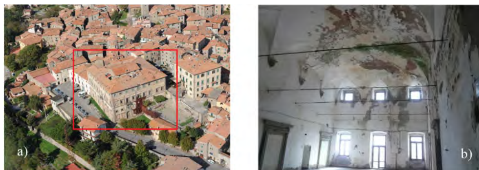
Figure 1. The Bourbon del Monte Palace in Piancastagnaio: (a) outside view; (b) inside view.
