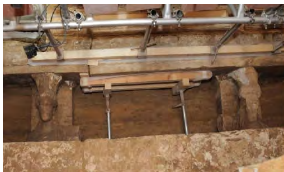
Figure 5. a. The Wall of the Maidens, as found, before the dismantling of the sealing wall, b. detail showing the vertical fracture in the west Maiden.
