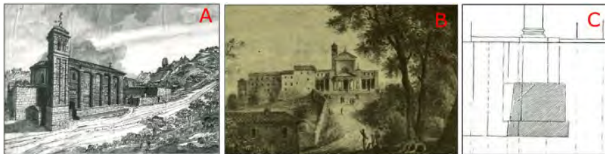
Figure 7. (A) The primitive church, showing the façade oriented toward the west, in a drawing of the 1793 by Giuseppe Fancelli. (B) Drawing of the new church of the 1828 (Osservanza Historical Archive). (C) Scheme of the underpinning work carried out on columns 5 and 6 of the right aisle (Osservanza Historical Archive, Section III, Vol. 1, doc. 15).
