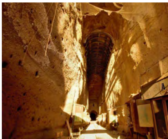
Figure 27. Western entrance of the Crypta Neapolitana in a recent photo. On the vault, the recently placed bolted steel arches.
