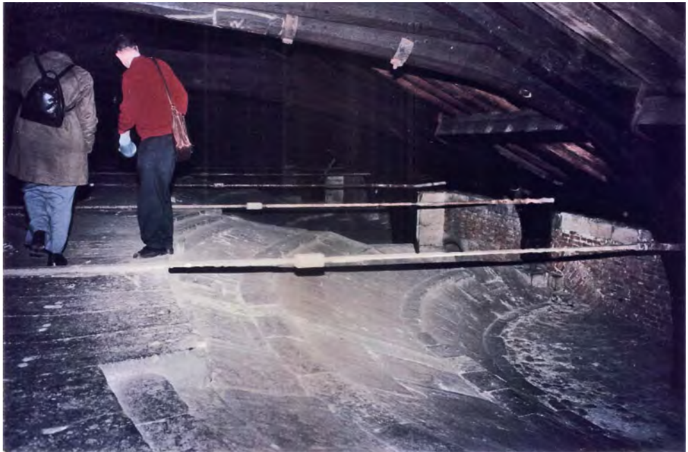
Figure 7. Extrados of the vaults of King's College Chapel. Cambridge, UK. Ph.: P. Smars, 2002.
