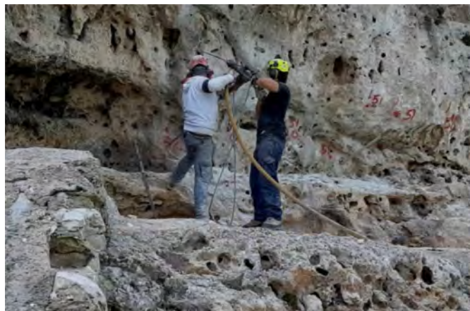
Figure 6. Favellato SPA technician preparing the holes in the limestone.
