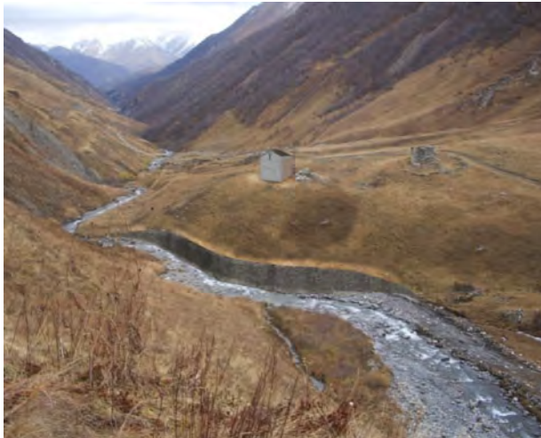
Figure 7. Proposed plan of restoration of the hill and the church after improving the riverbed and strengthening of its banks.
