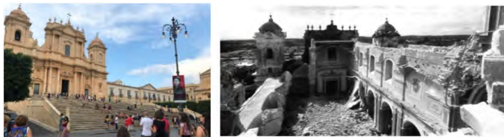
Figure 2. Noto cathedral. a) Front view of the building; b) Internal configuration after the 1996 collapse (Di Prisco et al. 2006).
