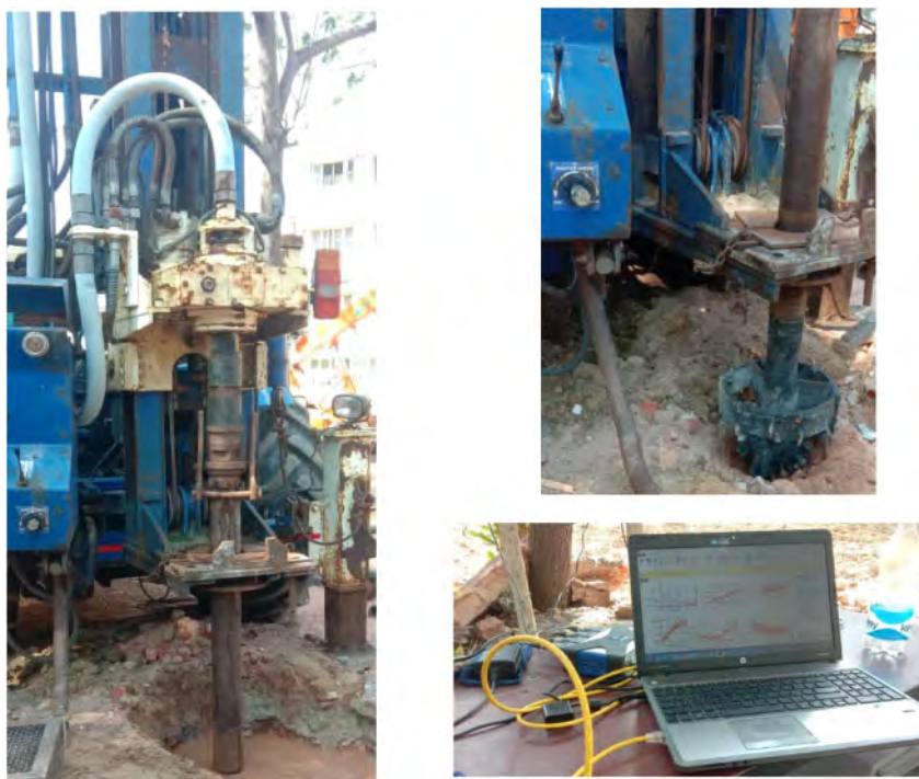
Figure 3. Pile driving operation at site.
