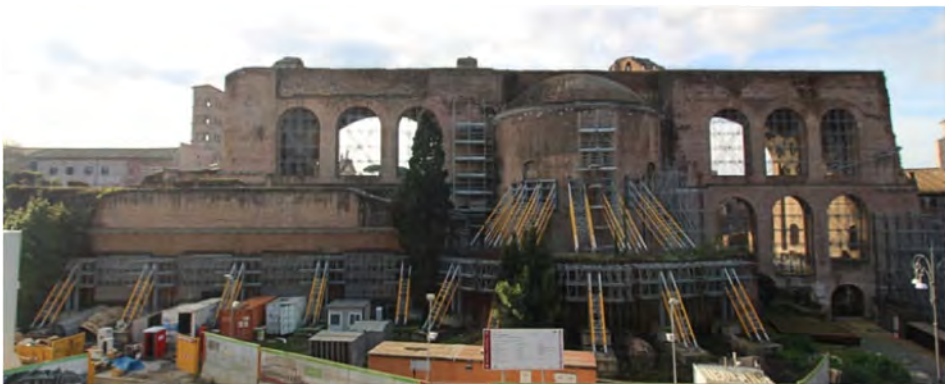
Figure 8. Temporary structural interventions installed on the Basilica.
