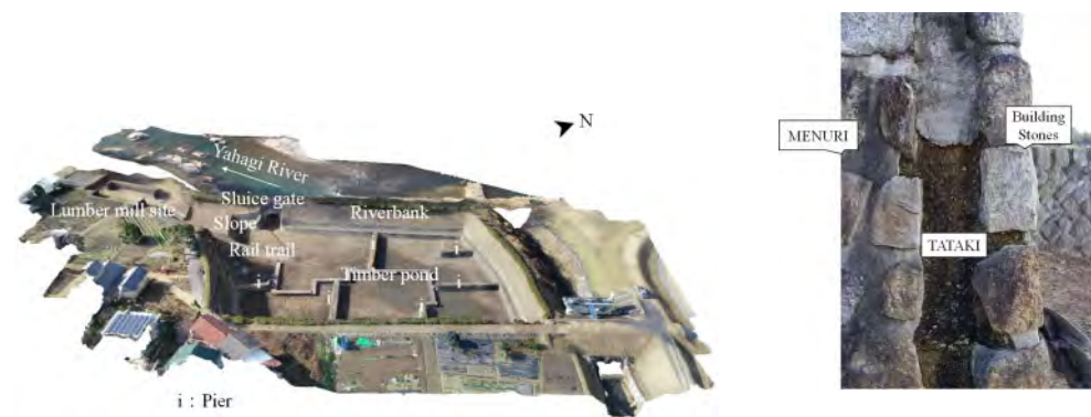
Figure 3. Characteristics of artificial stone structure.
