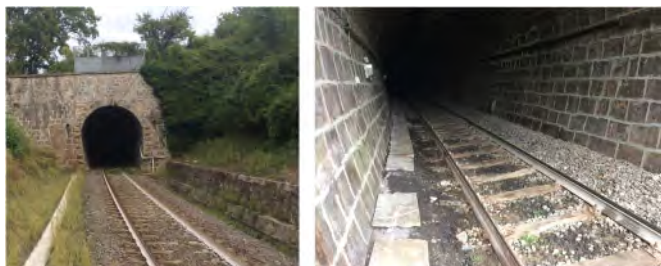
Figure 10. Galleria Sipicciano I: Photo of tunnel entrance ch. 7+228 (on the left) and photo inside the tunnel (on the right).
