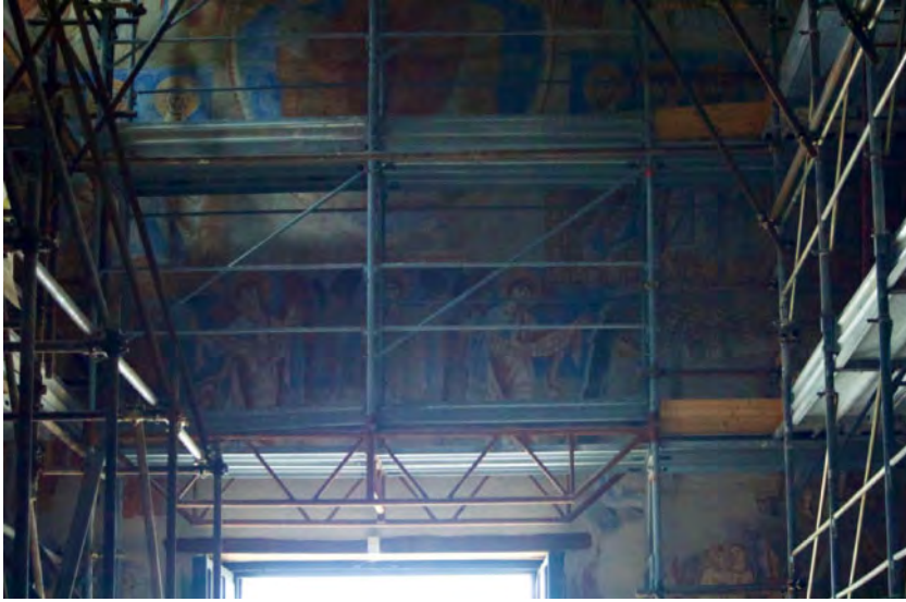
Figure 12. Recently carried out remedial works in the church.
