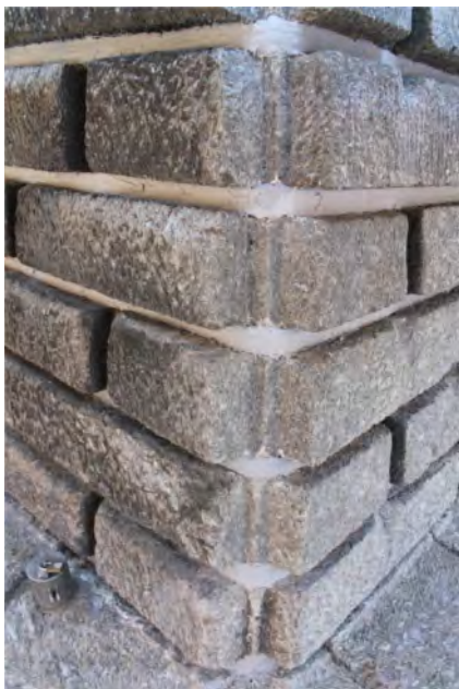
Figure 6. FRCM belting (A).
