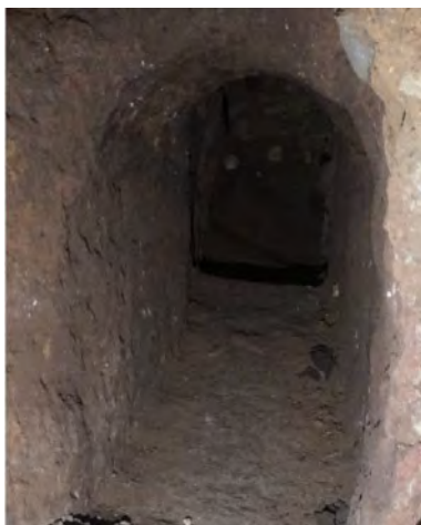
Figure 16. Unlined stretch of a tunnel excavated in the tierra café oscuro (modified after Lacombe et al. , 2020).
