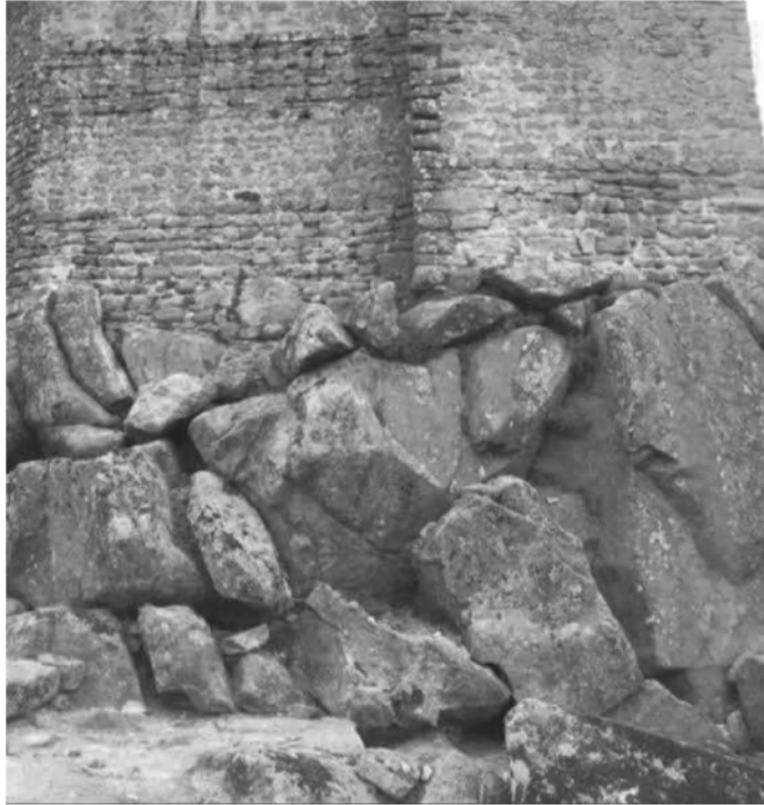
Figure 1. Examples of different degrees of weathering. To the right, moderately weathered granite (W3). On the left, slightly altered granite (W2).
