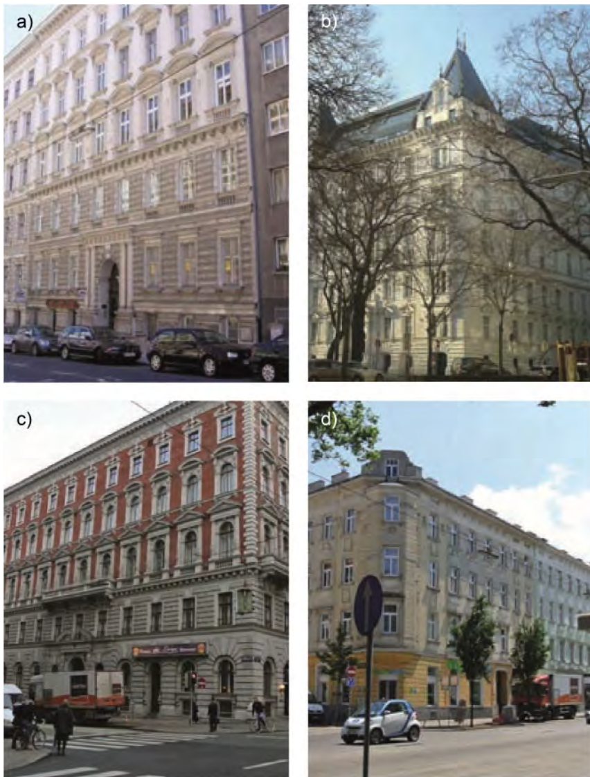
Figure 3. Overview of Gründerzeit buildings in the city of Vienna that undergone foundation soil treatment with expanding polyurethane resins.
