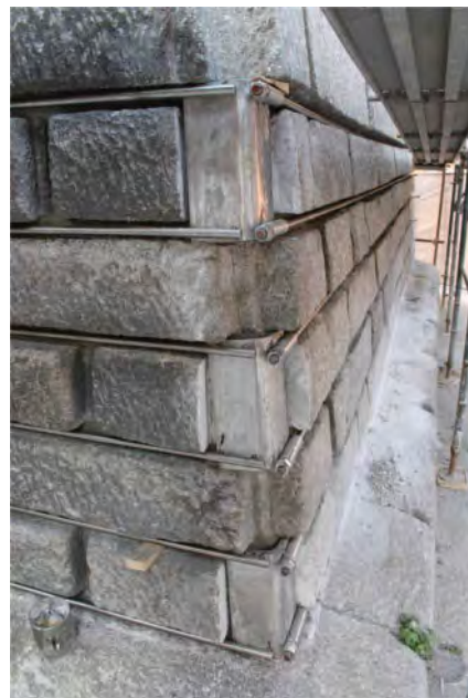
Figure 7. Post tensioned steel bars (B).
