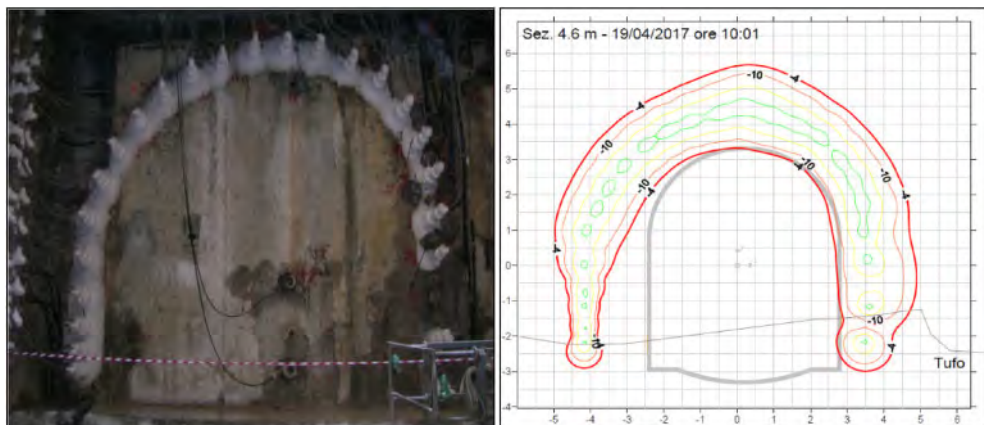
Figure 7. On the left, freeze and temperature pipes around the tunnel section; on the right, the isotherm contour map of the frozen body.
