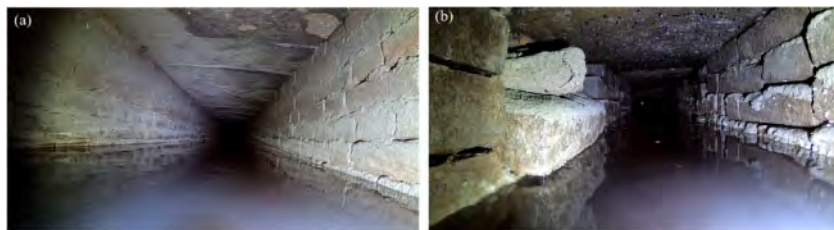
Figure 4. Inner view of two drainage conducts in S. Mark's square: (a) gatolo in good conditions, (b) gatolo in bad conditions.
