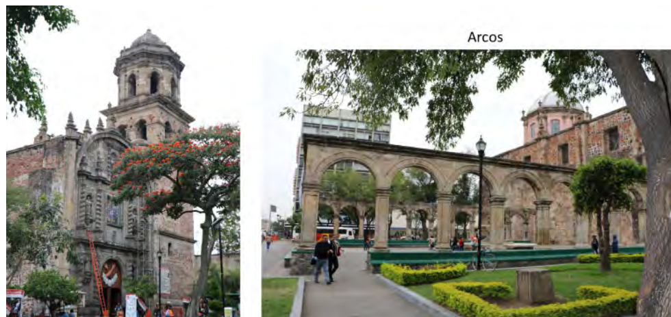
Figure 3. Left hand side: view of the main façade; right hand side: view of the reconstructed archway of the former cloister along the East side of the church.
