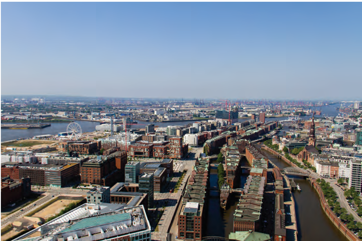
Aerial view of western HafenCity and Speicherstadt, Hamburg Germany. Photo by Thomas Fries (CC-BY-SA-3.0).
