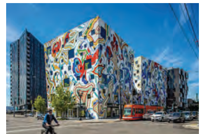
The Fair-Haired Dumbbell building, Central Eastside Portland OR, USA. Photo courtesy of Peter Eckert.
