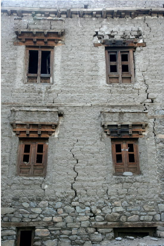
Fig. 4.32 (Left) Leh. Stone wall in the Old Town topped with an earth wall, both using timber lacing as crack stopper.
