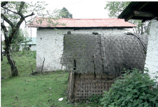
Fig. 4.12 Tawang. Arunachal Pradesh. Stone, clay and bamboo mats used side by side.
