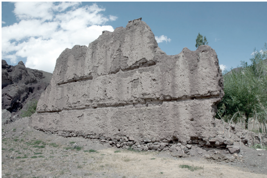
Fig. 4.43 Chigtan (Sgang). View from the south onto the ruins of a temple with notches of former timber lacing.
