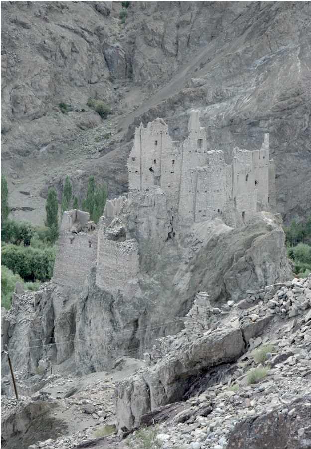
Fig. 4.40 Chigtan. Fortress made of rubble stone.
