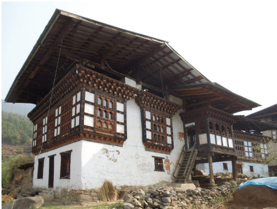
Fig. 4.11 West Bhutan. Located close to Paro along the road to the Tagtshang Monastery. Traditional rabsey construction. Photo: Roland Meingast 2016.
