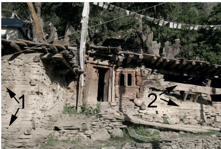
Fig. 4.75 Karla. In the picture left: dhol-maide construction (1). In the picture right (in ruins): kath-kuni construction (2).
