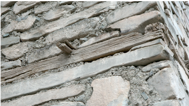
Fig. 4.41 Chigtan. Fortress. The stones are relatively flat. Corner half lap joint.
