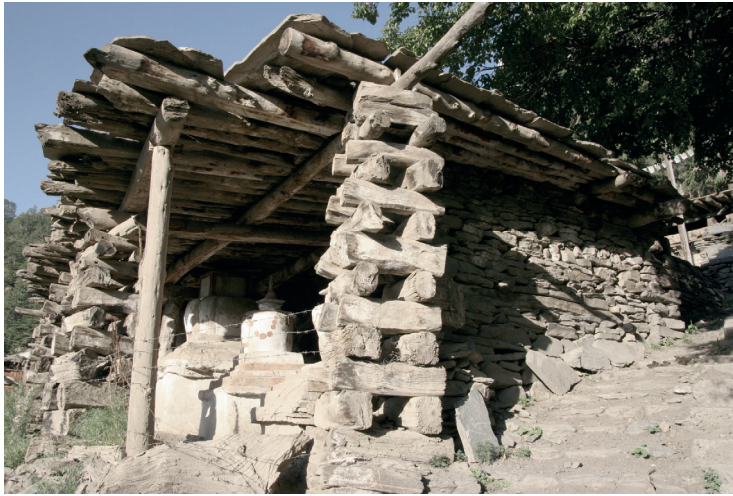
Fig. 4.73 Karla. Farque construction.
