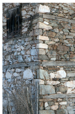
Fig. 4.19 Dolno Lukovo. Corner half lap joints.
