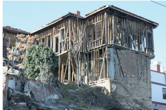
Fig. 4.8 Ankara, Turkey. Himiş structure on top of a solid ground floor.
