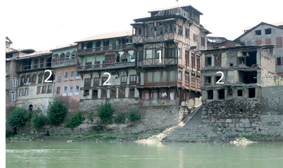
Fig. 4.10 Kashmir. India. Dhajji dewari (1) and taq (2) constructions along the banks of the Jhelum River.
