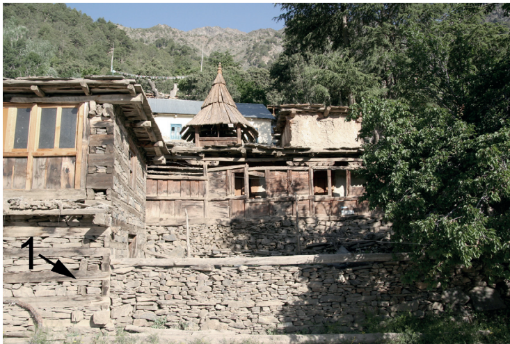
Fig. 4.74 Karla. In the picture left: kath-kuni construction (1).
