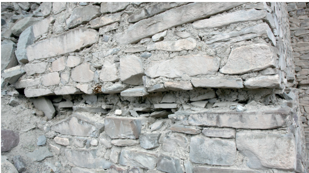
Fig. 4.42 Chigtan. Fortress. Timbers are laid on a plane stone level and covered by one layer of flat stones. Surrounding stones are pressed to the timber using a clay mortar.
