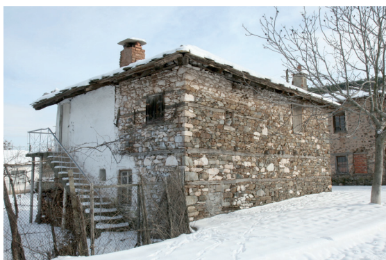
Fig. 4.18 Dolno Lukovo. Bulgaria. Stone walls with timber lacing.
