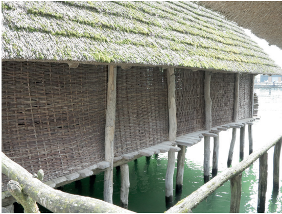
Fig. 4.1 Unteruhldingen. Germany. Pfahlbau Museum. Reconstruction of wattle walls of sunken structures of a lake dwelling settlement (975–953 BCE). The reconstruction of the technique is based on remaining imprints.
