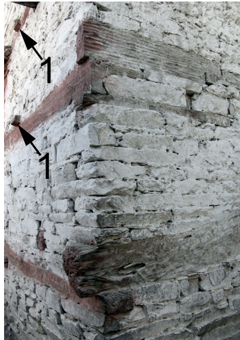
Fig. 4.85 (Bottom, right) Kanam. Kangyur Lhakhang. Dhol-maide construction.
