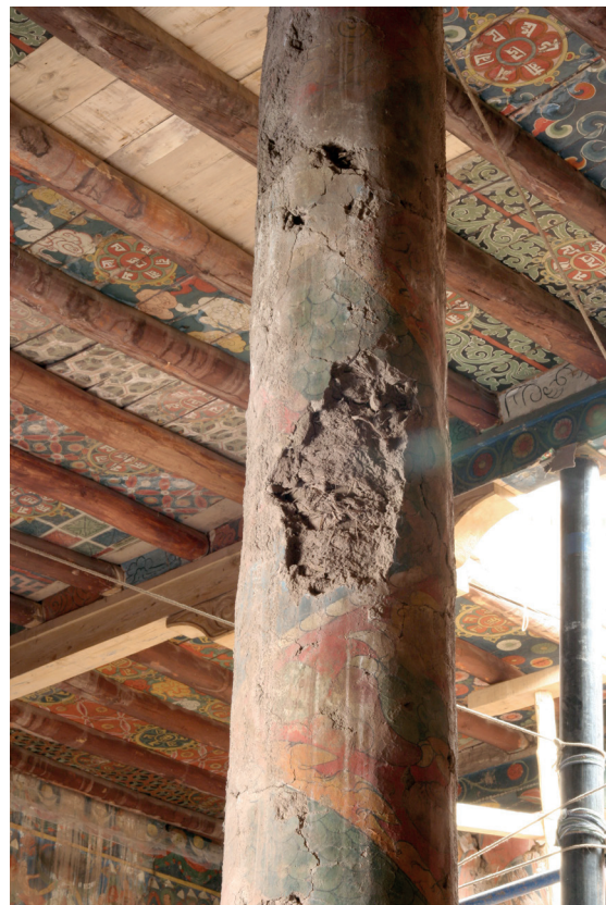
Fig. 3.3 (Left) Basgo. Maitreya Lhakhang. Ground plan and section. The ground plan shows the position of the round-shaped pillars. Fig. 3.4 (Right) Basgo. Maitreya Lhakhang. Damage at the plaster on a pillar.
