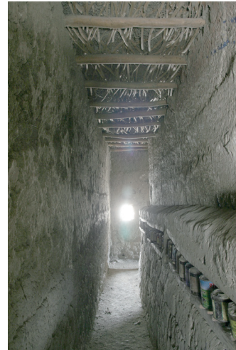
Fig. 4.63 Rangrik. Spiti. Temple walls made of rammed earth.
