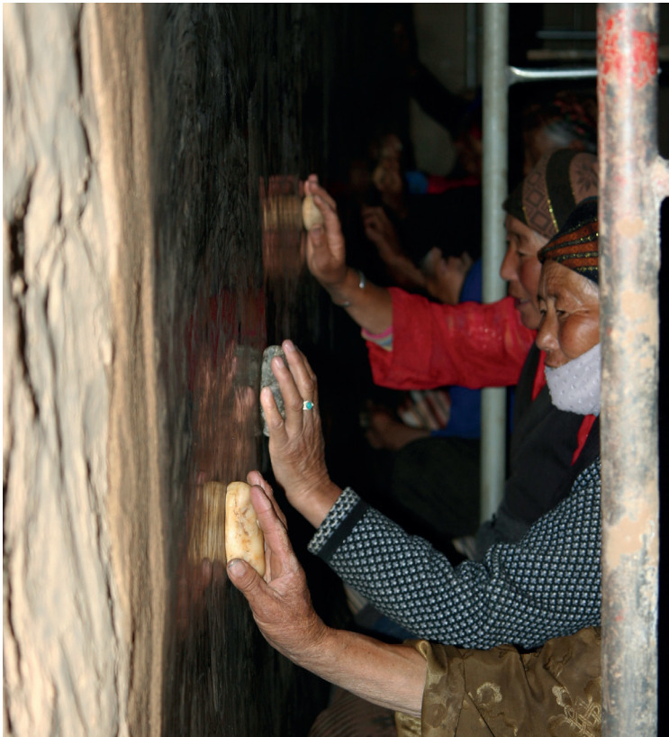
Fig. 2.3 Uru Katsel Temple. Women creating a shiny surface on top of the clay plaster by burnishing with round stones.
