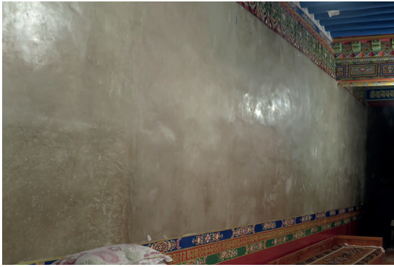
Fig. 1.15 Uru Katsel. Assembly hall. Shiny surface of a burnished clay plaster.
