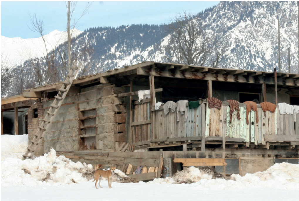
Fig. 4.48 Kalam, North Pakistan. Bhatar construction.
