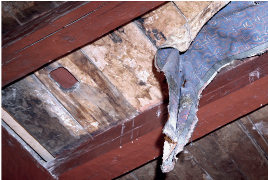
Fig. 1.13 Tabo. Tsuglagkhang. Painted textiles on wooden planks hewn with an adze.
