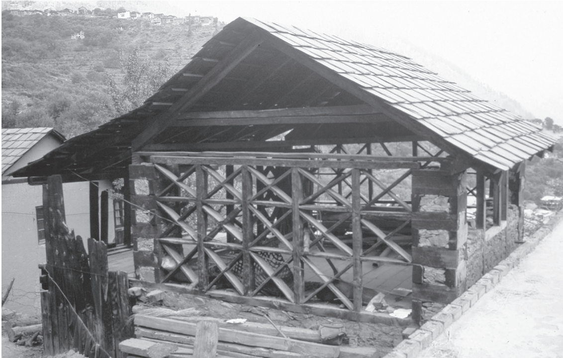
Fig. 4.98 (Top) Bharmaur. Chamba. Corners made as farque construction and the wall in-between as dhajji-dewari construction.
