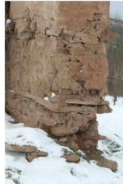
Fig. 4.17 Mandriza. Adobe brick walls with 'ladder'-like timber lacing.
