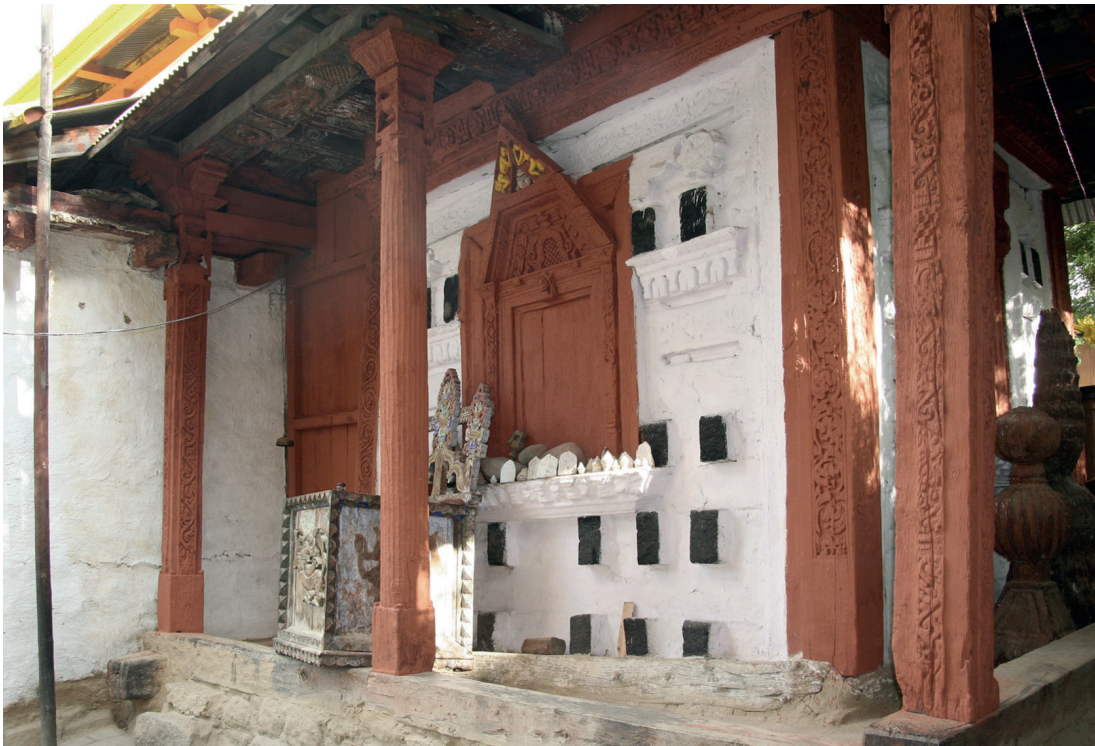
Fig. 4.91 Ribba. Middle Kinnaur. North facade.
