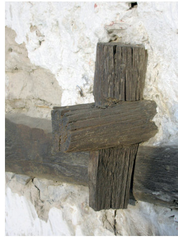
Fig. 4.37 (Top) Skurbuchan Khar. Timber lacing in the lower stone part of the wall.
