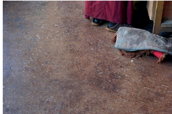
Fig. 1.14 Lhasa. Jokhang. Shiny surface of an oiled and burnished arga floor.
