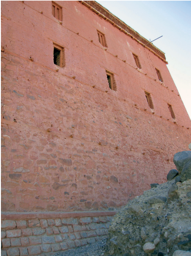
Fig. 4.35 Phyang. Two storeys with stone walls topped with two storeys of adobe brick walls. Timber lacing at floor level carries the floor beams. Along the facade runner beams are connected to halving joints.
