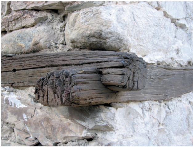
Fig. 4.37 (Top) Skurbuchan Khar. Timber lacing in the lower stone part of the wall.
