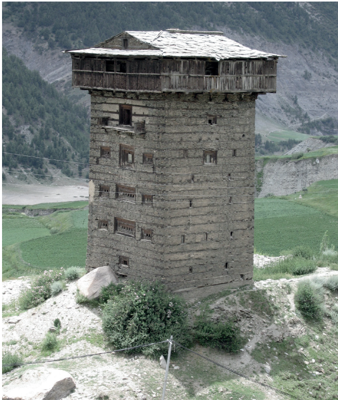
Fig. 4.60 Gondhla. Lahaul. Fortress tower.
