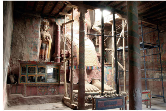
Fig. 1.16 Basgo. Maitreya Lhakhang. Painted clay plaster on round-shaped wooden pillars.
