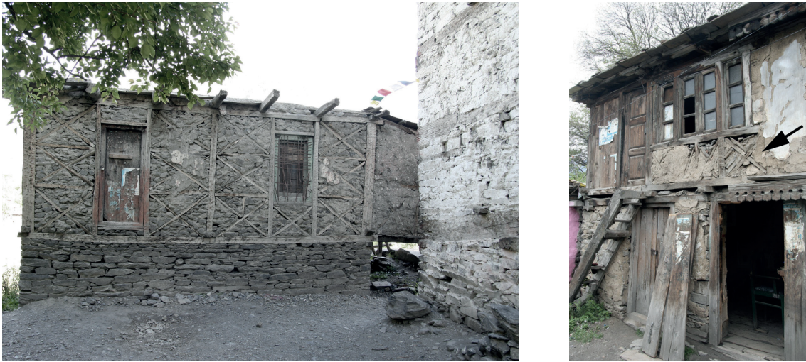
Fig. 4.86 (Left) Kanam. Dhajji-dewari structure attached to the Kangyur Lhakhang.
