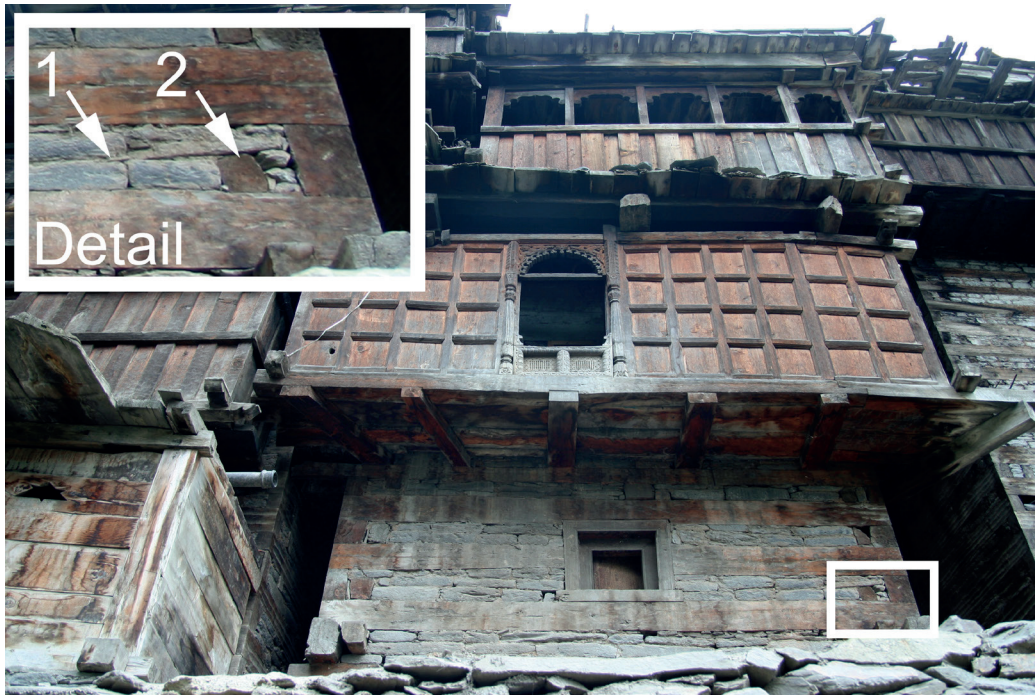
Fig. 4.80 (Top) Thangi. Middle Kinnaur. Verandas attached to the kath-kuni core of the building.
