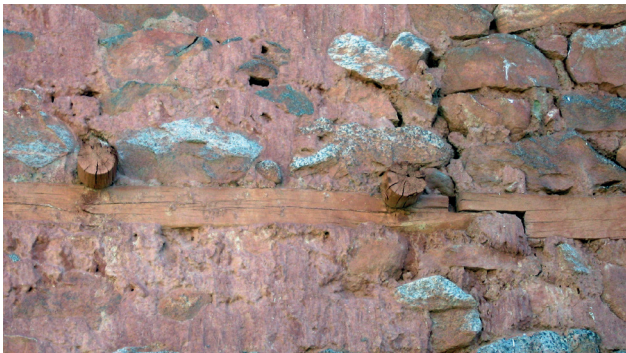
Fig. 4.36 Phyang. Floor beams are connected to the runner beams by lap joints.
