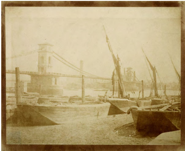
Figure 5.4 Hungerford Suspension Bridge, ca. 1845, taken by photographic pioneer Henry Fox Talbot.
