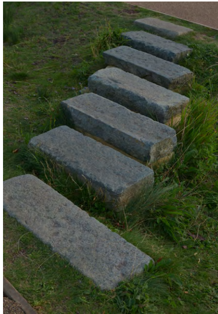
Figure 7.8 Granite kerbs reclaimed during clearance and demolition, reused as stepping stones in a playground in the east of Queen Elizabeth Olympic Park.
