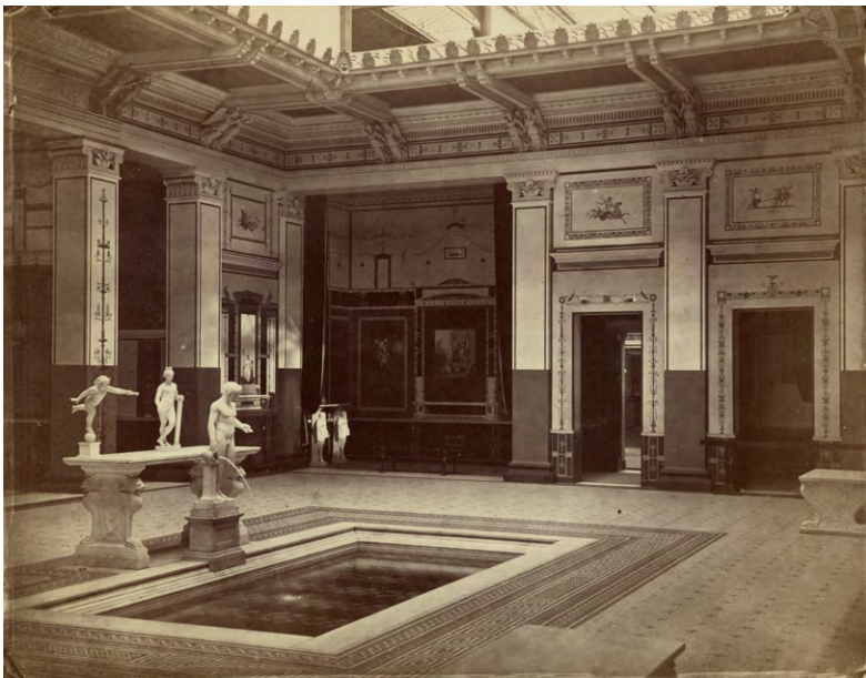
Figure 4.4 The interior of the Roman Court (ca. 1854), one of the Palace's Fine Arts Courts. The superstructure of the Palace can just be seen at the top of the image.
