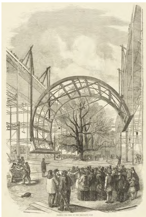
Figure 3.10 Raising the Palace transept’s wooden ribs in December 1850. Source: Reproduced from ILN 1850c. Courtesy of the National Library of Scotland. CC BY 4.0 .
