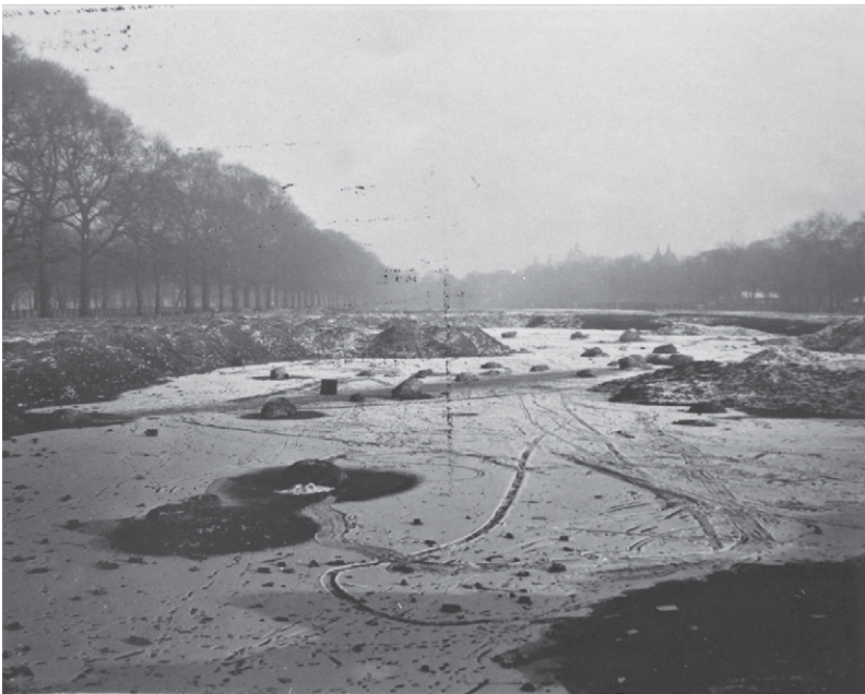
Figure 3.11 The concrete footings of the Crystal Palace in Hyde Park, uncovered during excavations for sand in 1939 and early 1940.
