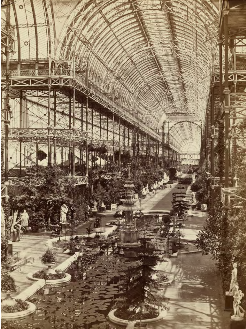
Figure 4.3 The nave of the Sydenham Crystal Palace in around 1854, showing its bayed structure; the Fine Arts Courts and other Departments were arranged along the sides.
