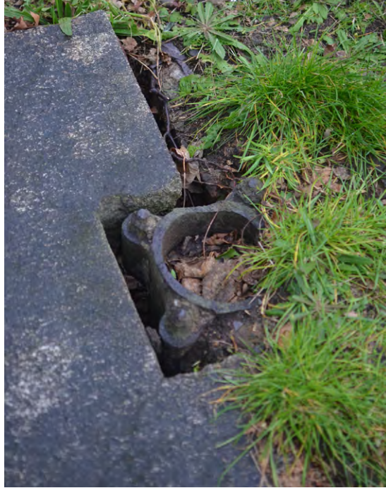
Figure 2.2 Scraps of a mega event: the socketed base of one of the Crystal Palace's cast-iron columns at Sydenham today. Source: Photograph by the author.
