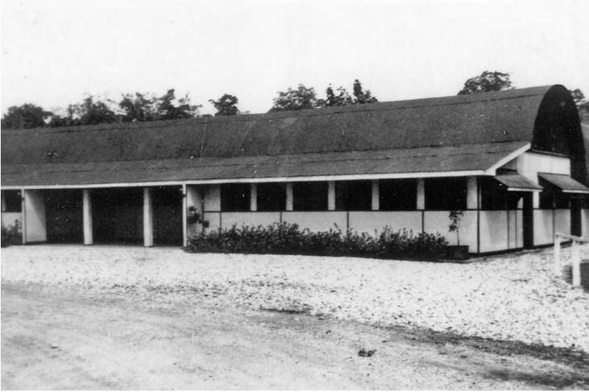
Plate 6.12 Honiara Police Station in 1952, constructed from a Quonset hut and scrap US Army materials.
