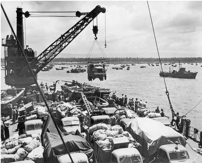
Plate 2.21 Unloading trucks at the lagoon at the mouth of the Lungga River.
