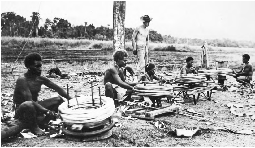
Plate 2.13 Solomon Islands Labour Corps unwinding copper wire for the telephone system, Camp Guadal, June 1943.
