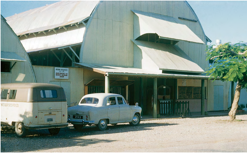
Plate 3.14 The Point Cruz Cinema in Mendana Avenue in the late 1950s. The cinema was constructed from Quonset huts with open sides to enhance air flow. Source: BM, Patrick Barrett Collection.
