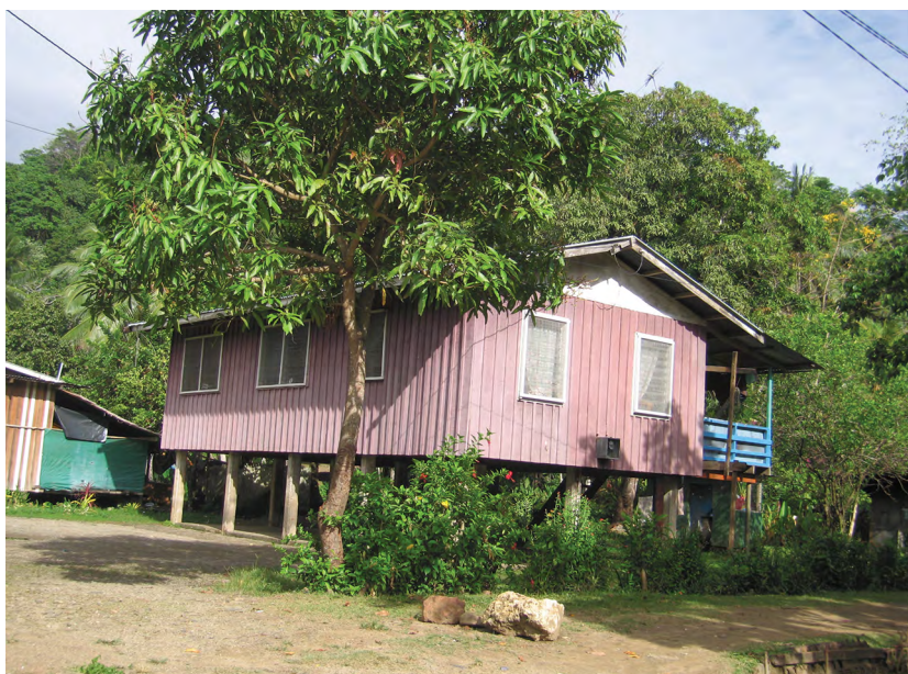
Plate 5.11 A Housing Authority home at White River, 2008.
