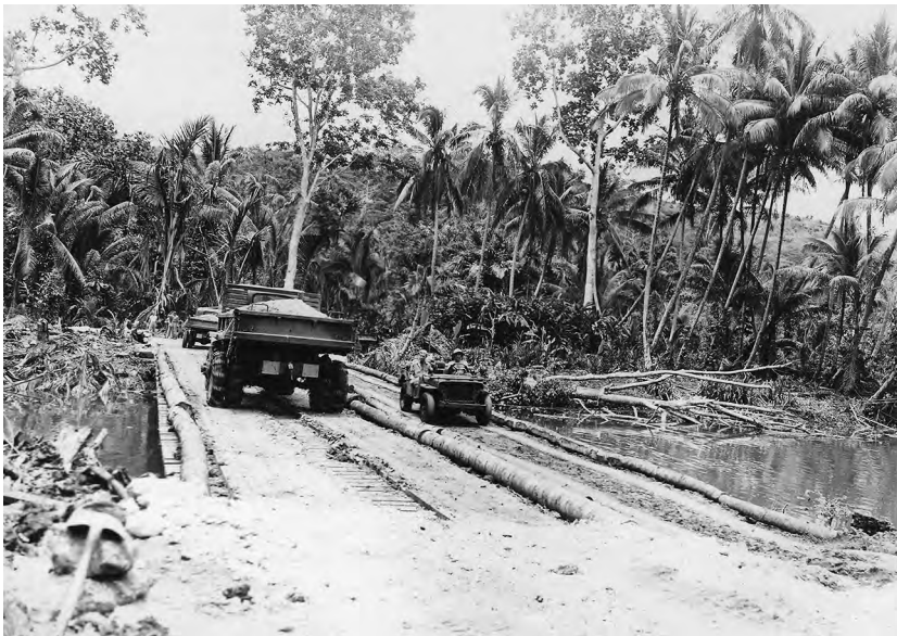
Plate 2.6 The Mataniko River vehicle bridge built by the Americans, 1943.
