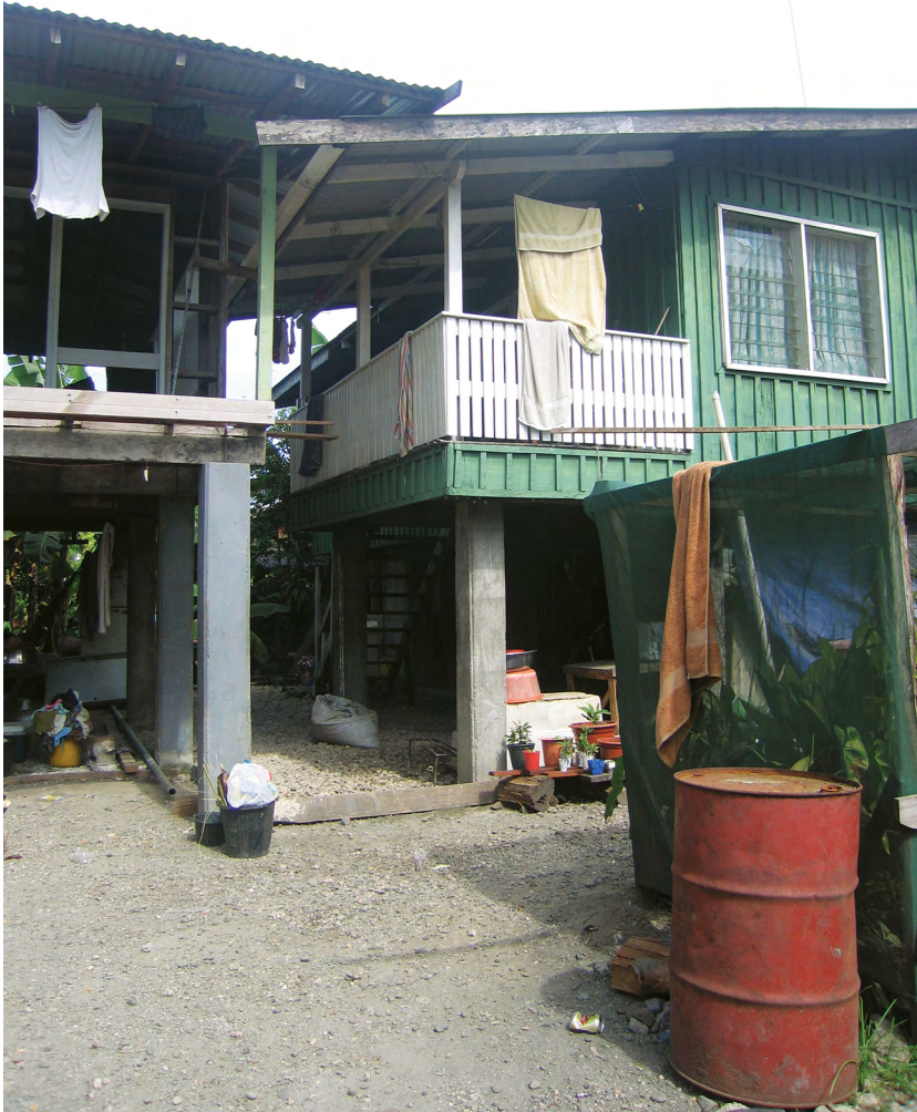
Plate 10.2 Hybridity: Neighbouring houses at Fishing Village are often built close together.
