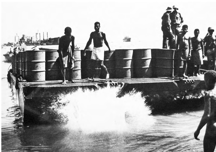
Plate 2.11 Solomon Islands Labour Corps unloading fuel drums at Lungga Beach, March 1943.
