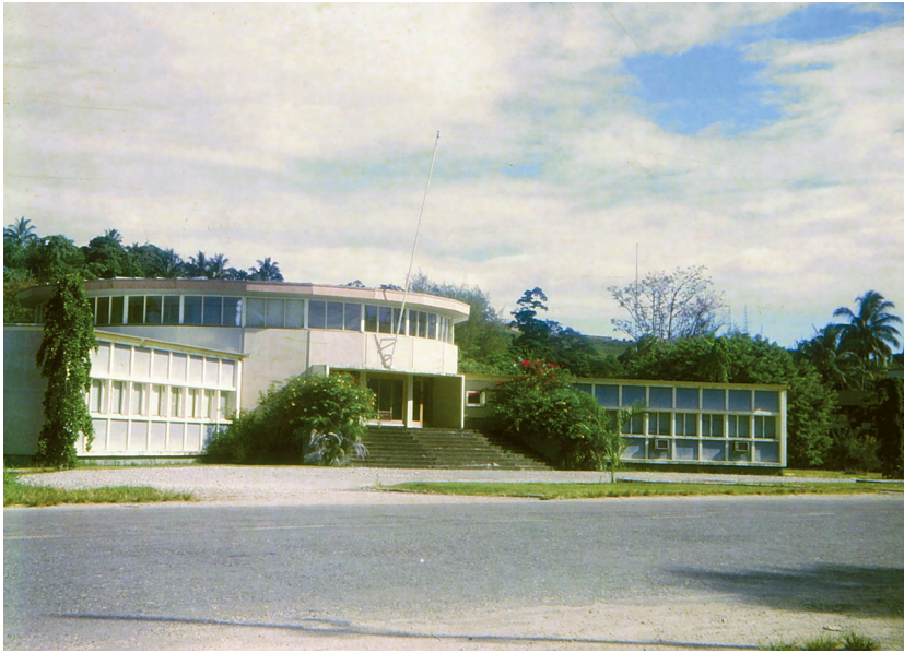
Plate 6.1 The WPHC High Court building was built in 1964.
