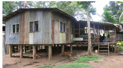
Plate 5.17 The original 1970s Toa Te`e house at Kobito 2 had ripple-iron walls as well as an unlined roof.
