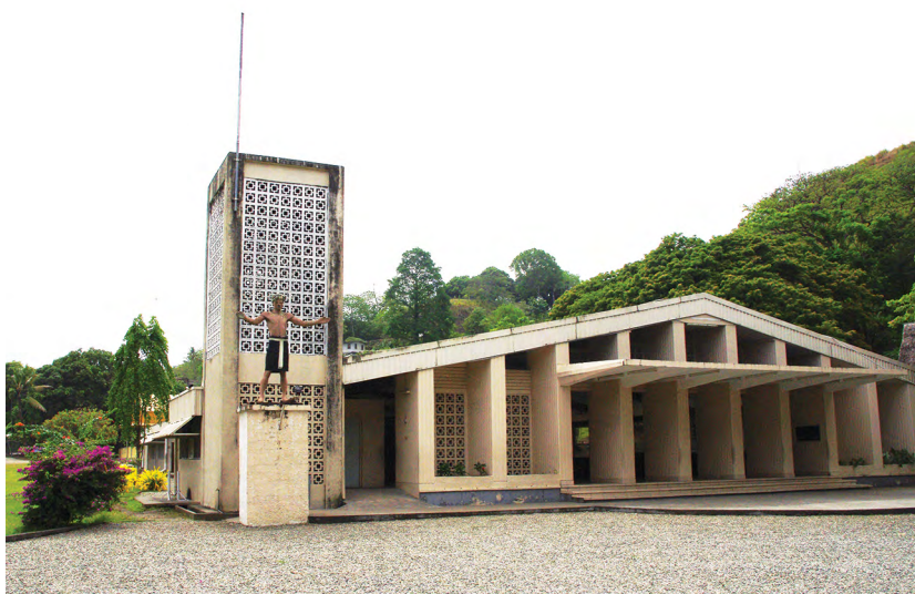
Plate 7.2 St Barnabas' Anglican Cathedral, 2017. It was built between 1968 and 1969.
