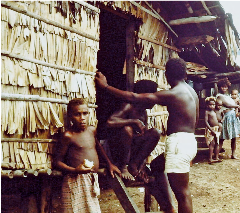
Plate 5.14 The first houses at Kobito 2 were built from local materials. This photograph is from 1968.
