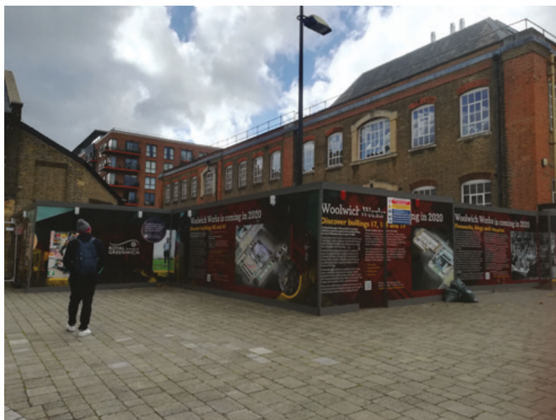
Fig. 2.6 ‘Woolwich Works’ under construction, Royal Arsenal. (Photo taken by the author, 10 September 2021.)
