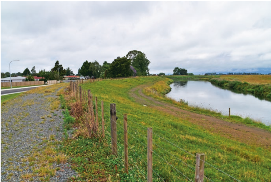
Photo 2.2 Rebuilt Flood levee in Edgecumbe, New Zealand. (Credit: Meg Parsons)
