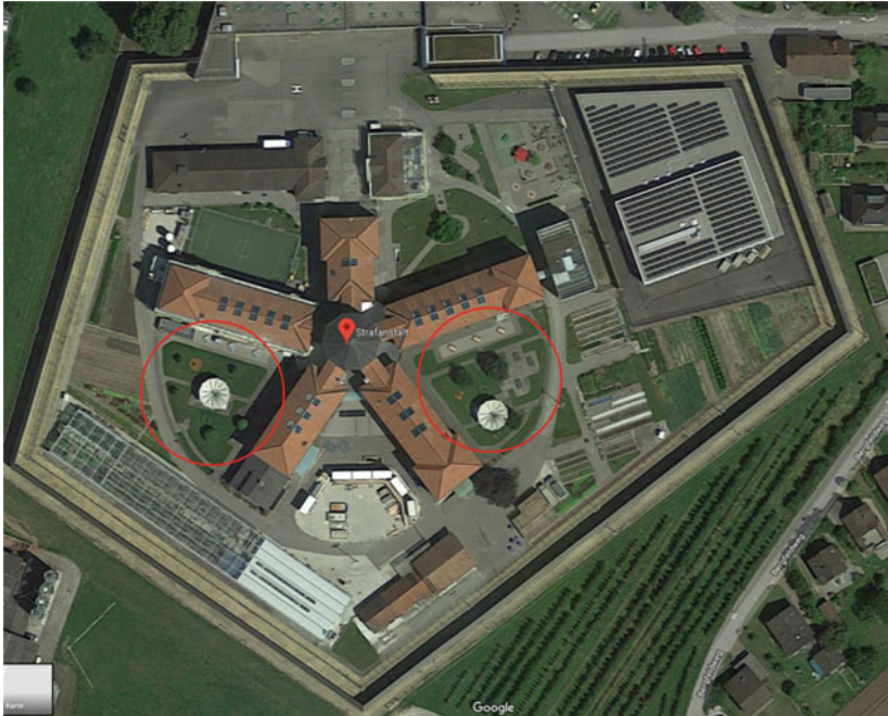
Fig. 6.1 The courtyards in the Strafanstalt at JVA Lenzburg (Source Google Maps)
