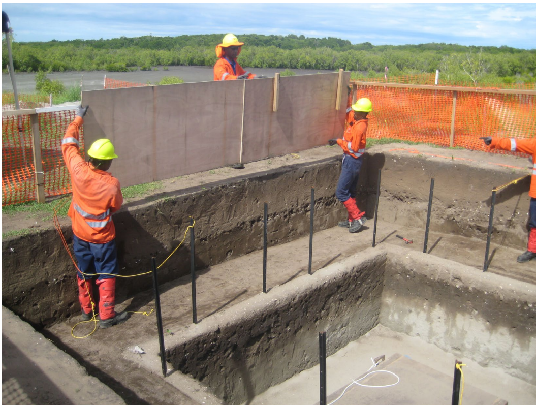
Figure 2.11. Removing shoring after excavation of the outer ring of excavation squares, Tanamu 1. The central trench (Squares A and B, bottom-right of photo) is covered by a wooden lid.
