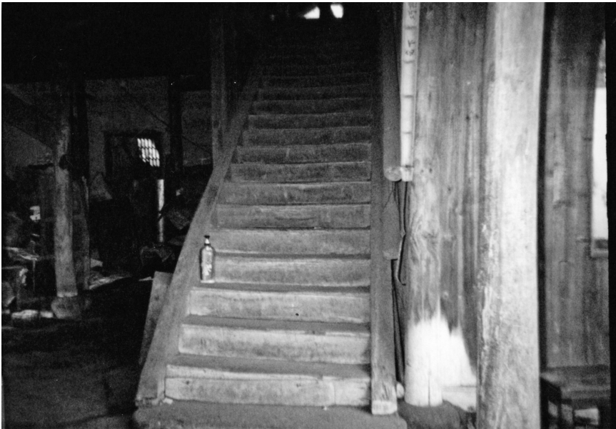
Figure 0.8 Staircase. Photo by Ms. Luo Yan.
