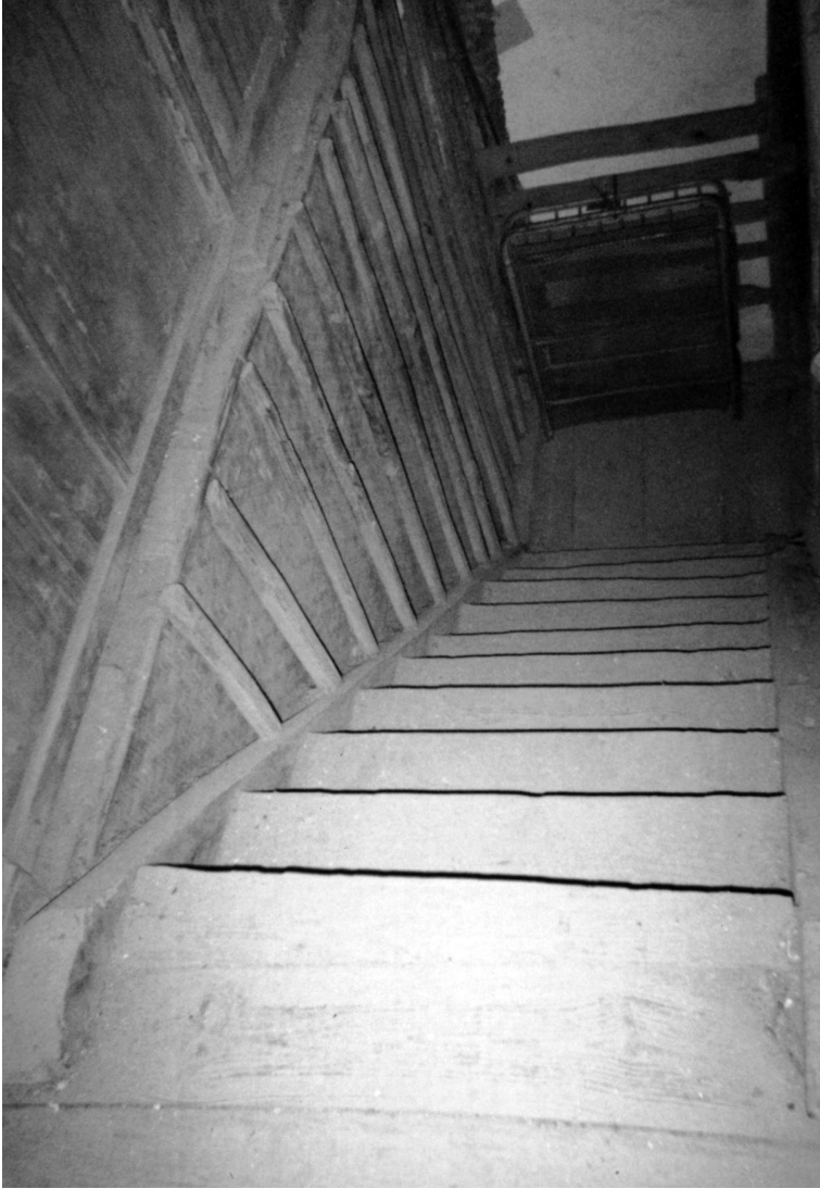
Figure 0.9 Staircase. Photo by Ms. Cheng Jv.
