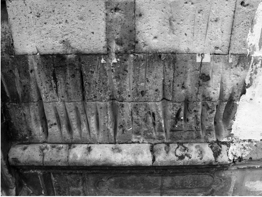
Figure 4.10 The deep grooves on the brick façade of Degengju were the result of children of many generations playing sliding coins.
