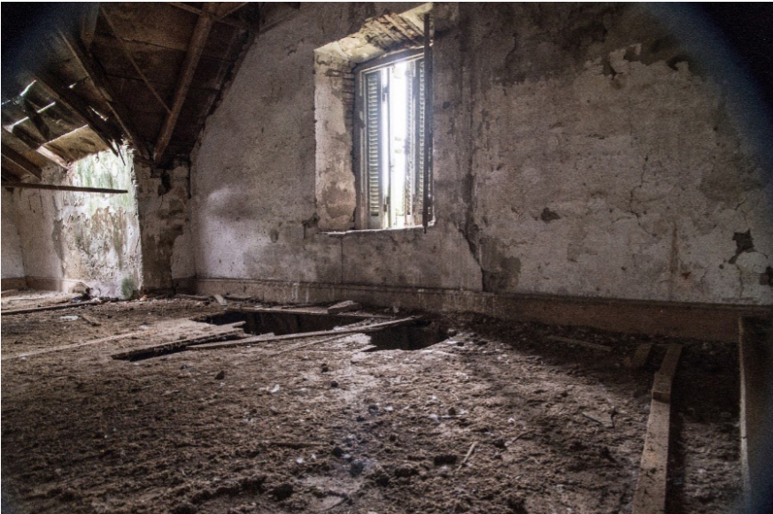
Photo 12. Old abandoned estancia house.
