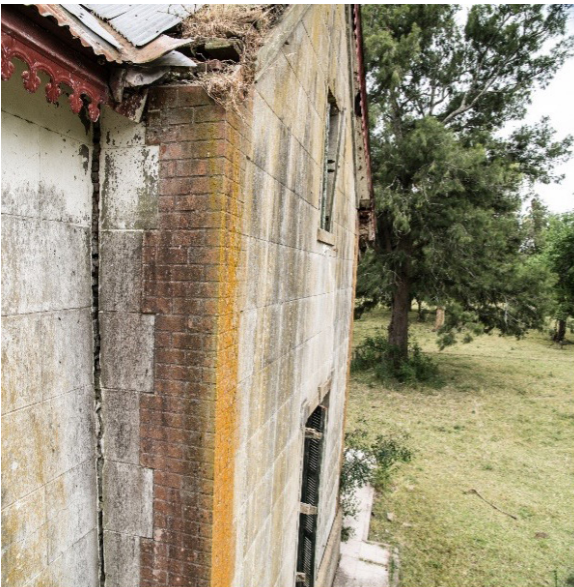
Photo 7. Old abandoned estancia house.
