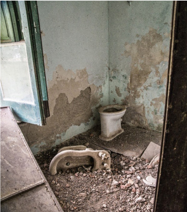
Photo 9. Old abandoned estancia house.
