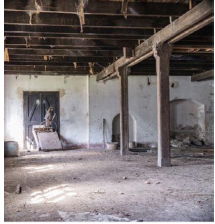
Photo 16. Old abandoned building that served as a ranch warehouse.
