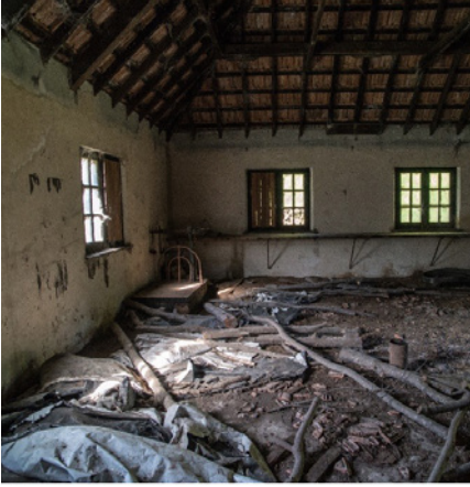
Photo 15. Old abandoned building that served as a ranch warehouse.
