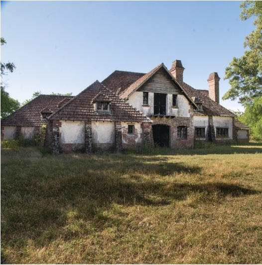
Photo 13. Old abandoned building that served as a ranch warehouse*
