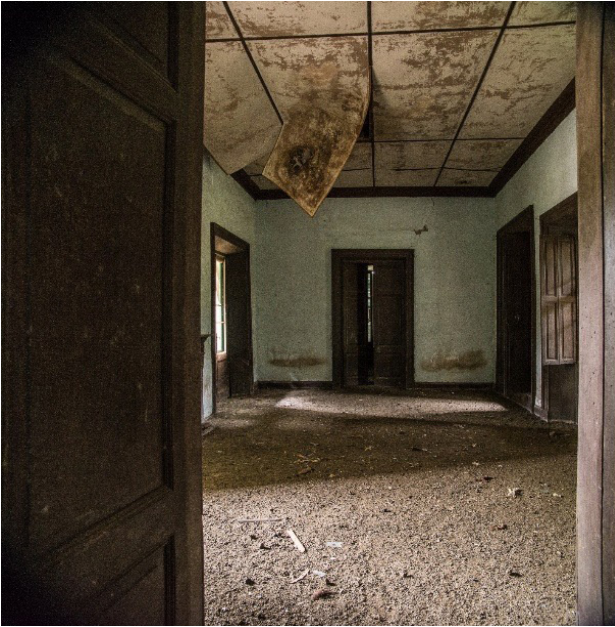
Photo 8. Old abandoned estancia house.
