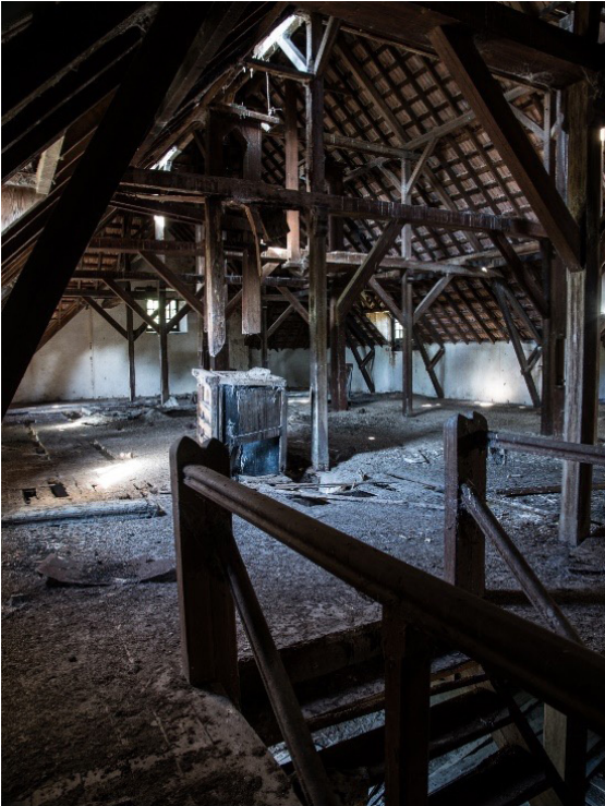
Photo 17. Old abandoned building that served as a ranch warehouse.
