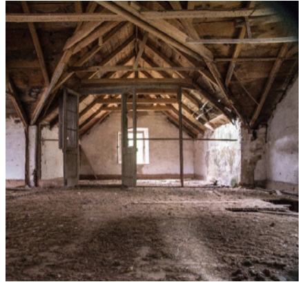
Photo 11. Old abandoned estancia house.
