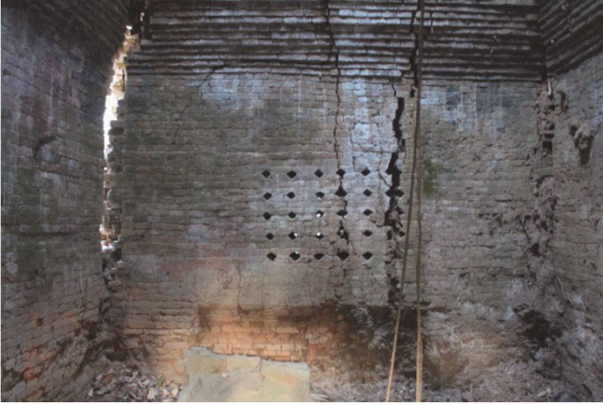
Fig.6: Interior view of Hiraṇyaruṇi's library at Phnom Khna taken in February 2013, showing the lozenge-shaped holes in the sides of the building. Photo: Julia Estève
