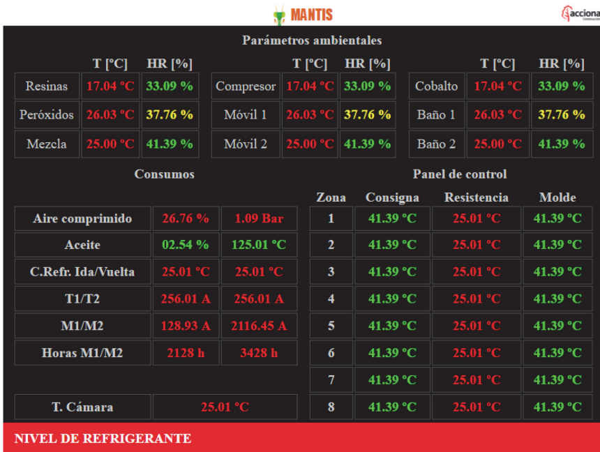
Figure 7.16 Local HMI. PC, Tablets, mobile devices.
