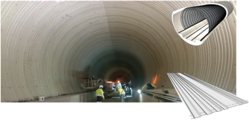
Figure 7.11 Waterproofing the Pajares tunnel in Asturias, Spain.
