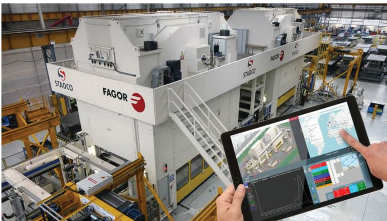
Figure 7.37 Predictive maintenance HMI platform.
