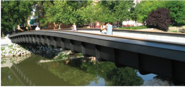
Figure 7.13 Pedestrian bridge in Madrid (Spain).
