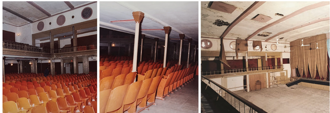
Fig. 05. The theatre auditorium at an elevation of 3.30 m, with the tribune supported by slender cast-iron columns (Photo archives of the Soprintendenza dei Beni Culturali ed Ambientali of Catania, to the left and centre, photos n. 82962 and 82977, taken in 1987 by Salvatore Lombardo - Project Archive, Matteo Arena Fund, University of Catania, SDS Architecture, Syracuse).
