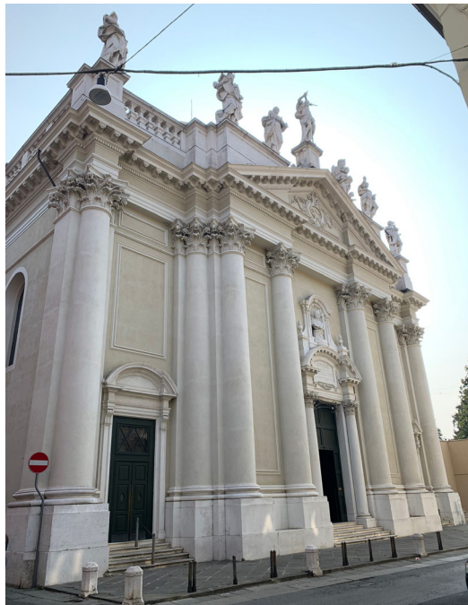
Fig. 04. The church of Saints Nazario and Celso in Brescia (photograph of M.Pontoglio Emilii).
