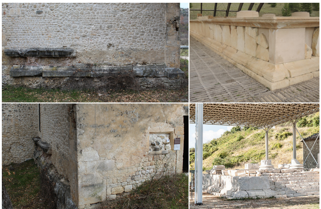
Fig. 02. View of the church's left front with the remains of the temple and typological comparisons in the Abruzzo region (photo by authors).
