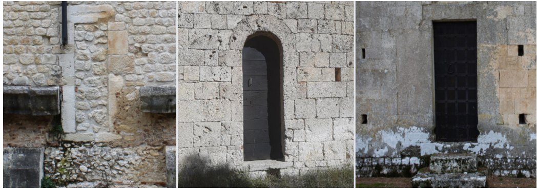
Fig. 03. View of the walled door on the left front of the Santa Maria della Vittoria church and comparisons with others in the L'Aquila area (photo by authors).
