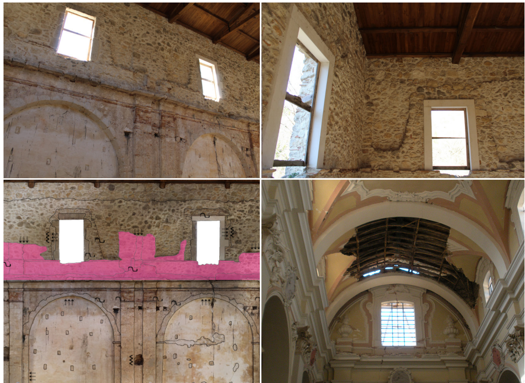
Fig. 04. Top: detailed images of the masonry of Santa Maria della Vittoria , bottom left: archaeological analysis and right: typological comparison with the San Domenico church in L'Aquila. (images and graphic elaboration by the authors).
