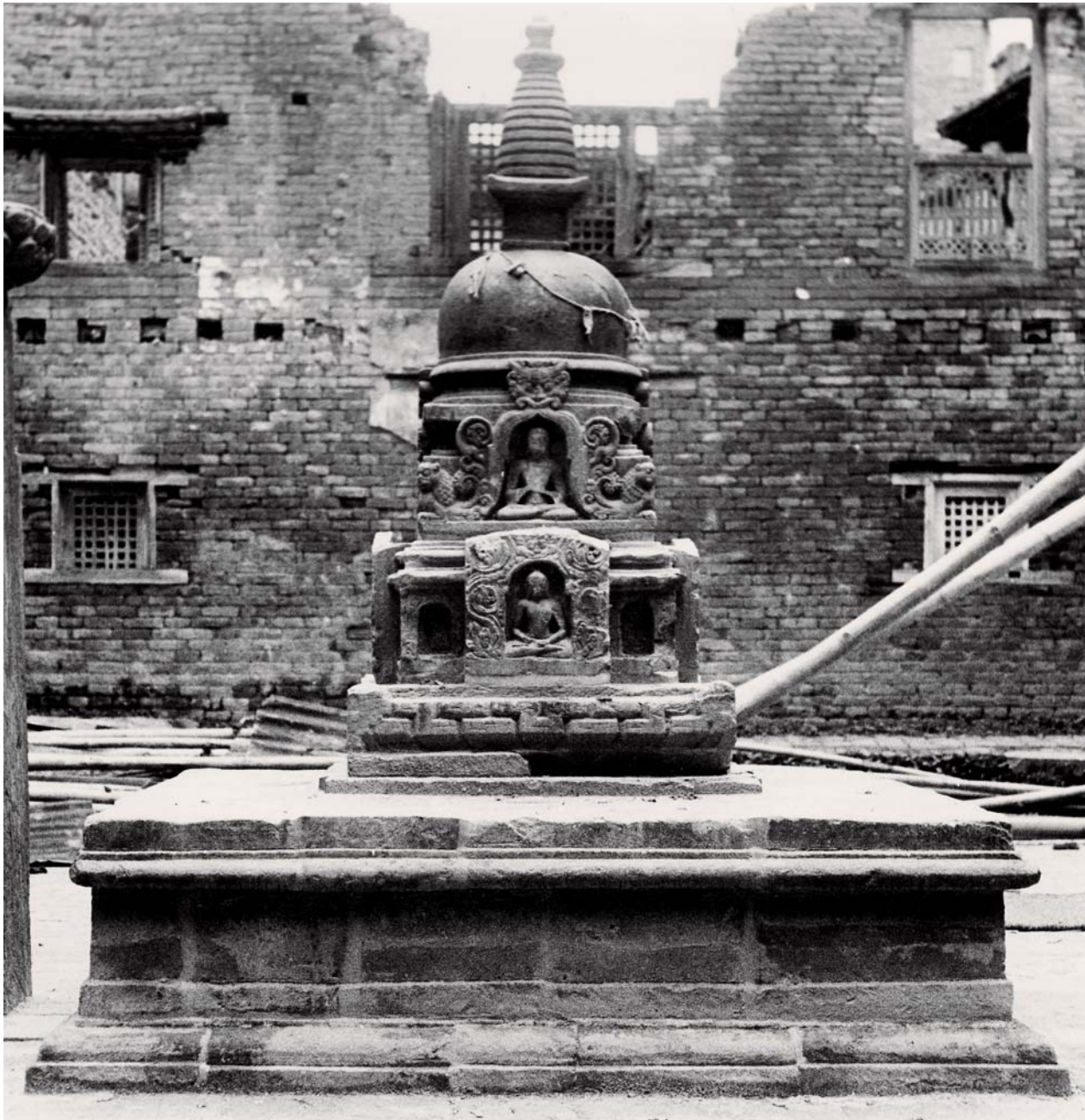
Vābhā Licchavicaitya, 7 th century, elevation east after dismantling and reconfiguration. The concealed rock motifs were lifted and the platform reinstalled in its 17 th -century dimension. Photograph by Niels Gutschow, August 1993
