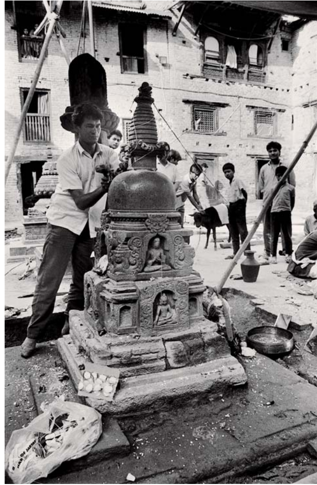
Vābhā, the Jivaninyāsa Pūjā The stone mason initiates the dismantling of the caitya . A rope is tied to the pinnacle of the caitya and the other end to the tail of a cow. A short jolt indicates the beginning of the dismantling. Photograph by Nutandhar Śarmā, May 17, 1993.
