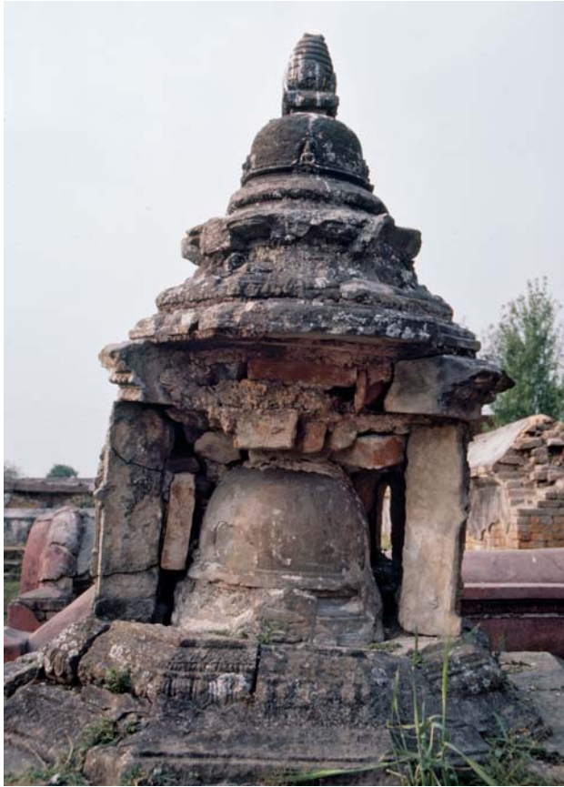
Bhaktapur Octagonal early 18 th -century Śikharakuṭācaitya on a triple- stepped platform at the eastern edge of Siddhapūkhū. The structure on the verge of collapse, its three southern niches already disintegrated. Based on the specific profiles of the drum; the enshrined object is datable to the 8 th century. Photographs by Niels Gutschow, June 11, 1987
