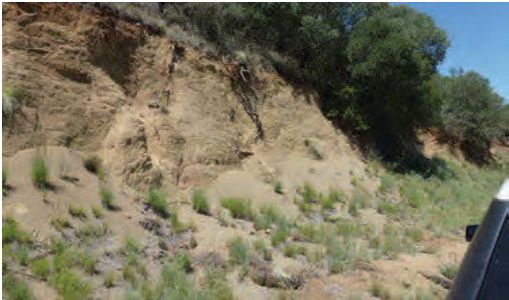
Figure 4.1. Deep weathering on dolerite exposed in a road cutting in the west-central Free State Province, South Africa.
