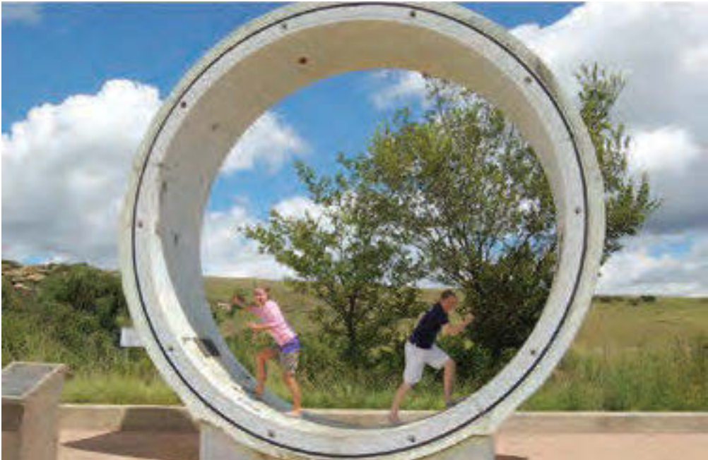
Figure 4.5. Lesotho Highlands Water Project monument at the Ash River outfall: a concrete lining with coarse dolerite aggregate was used to stabilise the sandstone and basalt transfer tunnels that weathered rapidly on exposure after drilling.
