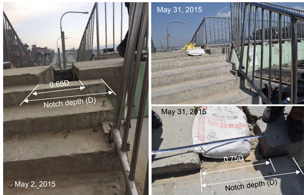
Fig. 9 Pedestrian overpass over Kathmandu-Bhaktapur Road at Kausaltar ( 27^{\circ}40.475' \text{ N } 85^{\circ} 21.865' \text{ E} ) (based on Konagai et al. 2015): the northern pier was on an outward tilt, causing the joint between the pier and the deck to open up
