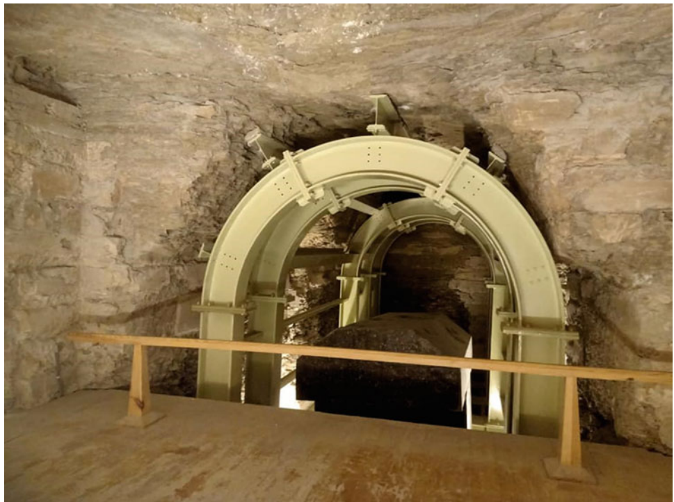
Fig. 9 A typical view of the metallic support structures installed at the burial chambers of the Serapeum in Saqqara
