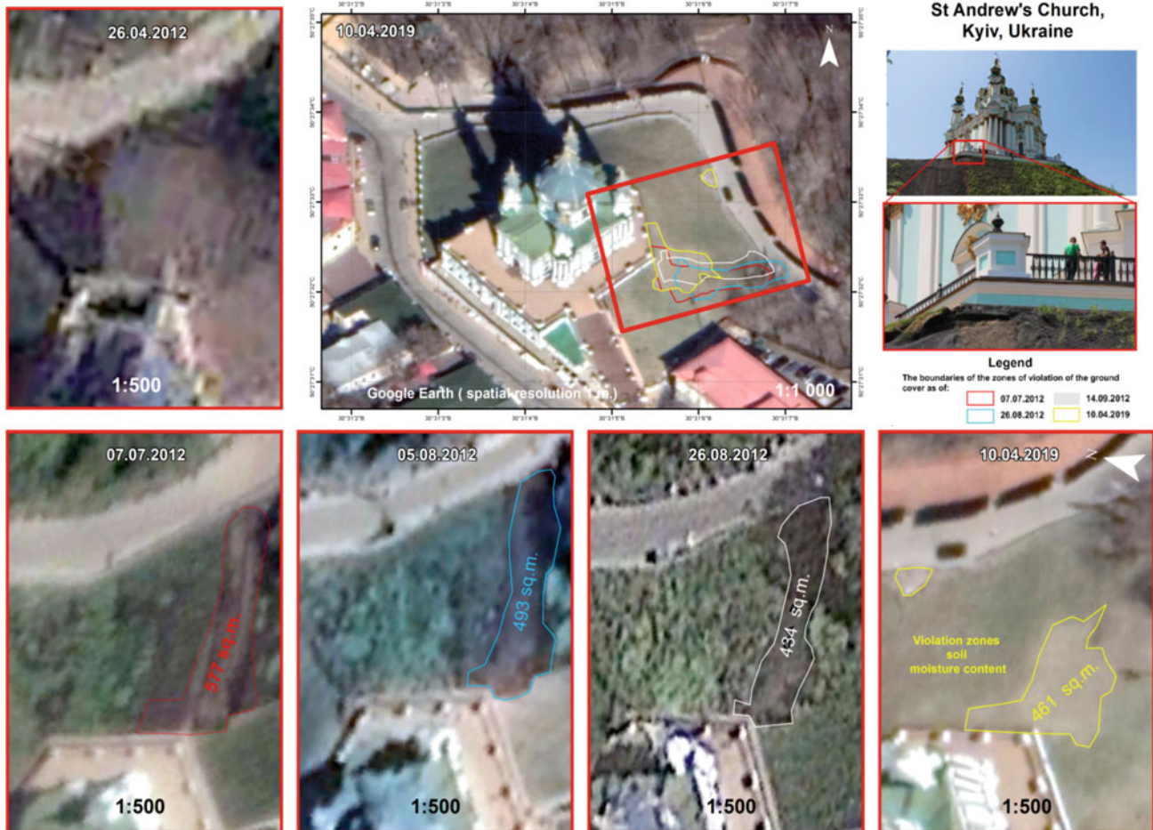
Fig. 8 Identification of landslide-hazardous areas according to Google Earth
