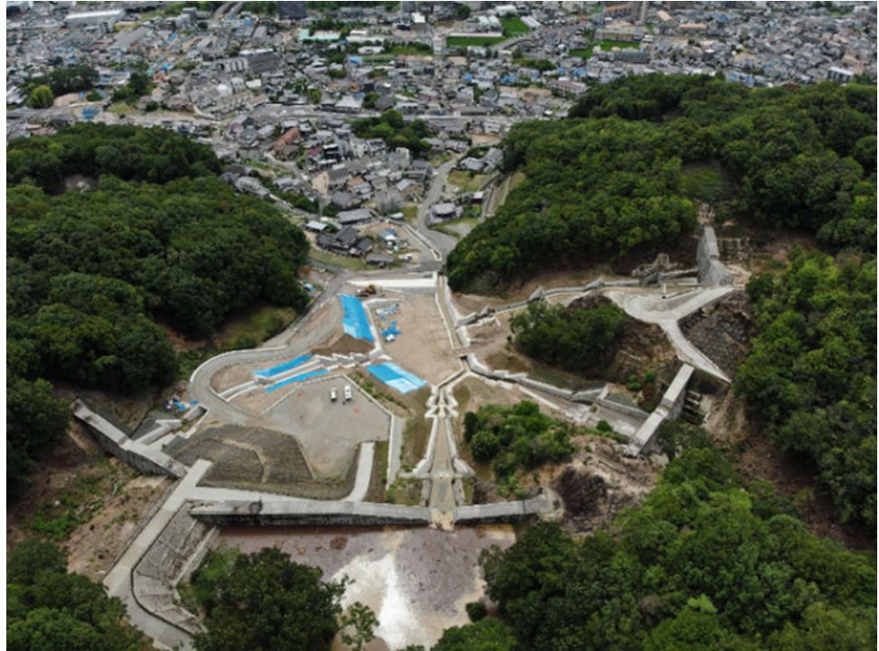
Fig. 26 Sediment capture behind a Sabo dam in the catchment 1-9-299 in Fig. 25 (Modified from source: Hiroshima West Mountain Range Sabo Office, MLIT 2019)
