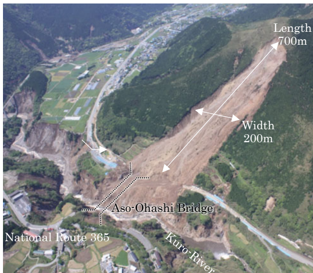
Fig. 10 A slope failure induced by the mainshock near the Aso-Ohashi Bridge (Modified from the Kyushu Regional Development Bureau, MLIT 2016)
