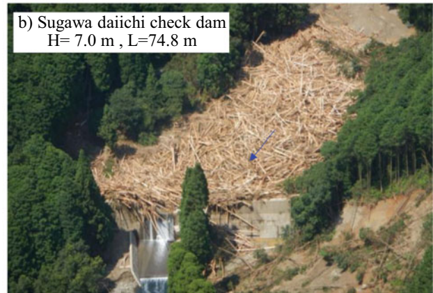
Fig. 2 a Typical erosion at Shirakitani river. b Catchment of driftwood by check dam (JGS 2018)
