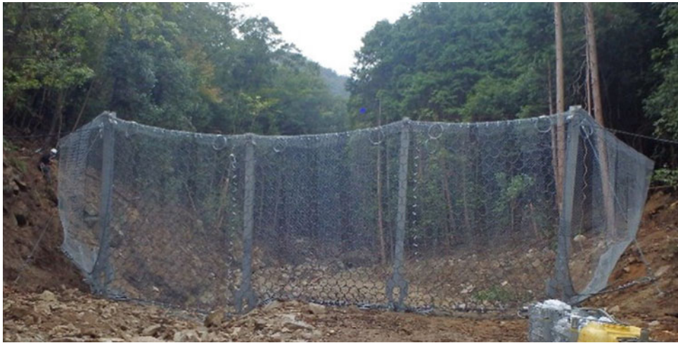
Fig. 24 Wire net barrier to capture sediment (Hiroshima West Mountain Range Sabo Office, MLIT 2019)
