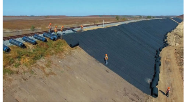
Fig. B.2 Geosynthetics used to stabilize a slope by interacting with vegetation root structures
