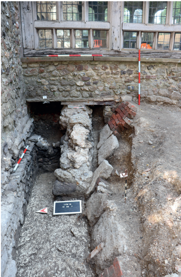
Fig 33. Foundation of north nave wall, western section. Photograph: authors.
