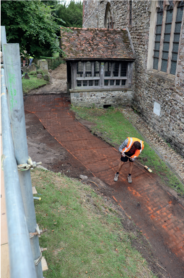
Fig 10. Former brick path to south porch revealed under its tarmac successor. Photograph: authors.
