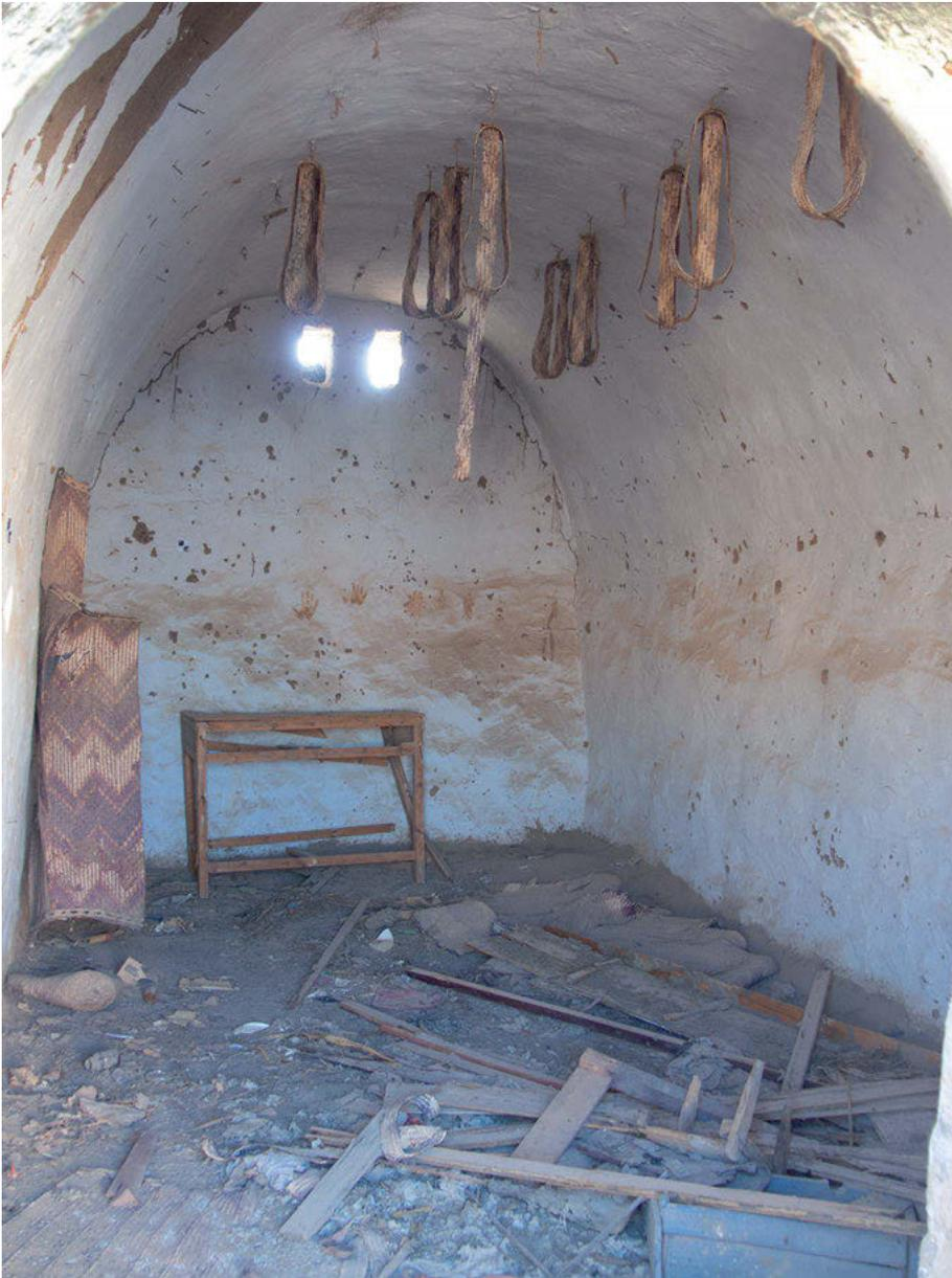
**Fig. 8:** Ventilation openings near the ceiling of a room in an abandoned Nubian house on Biggeh Island.
