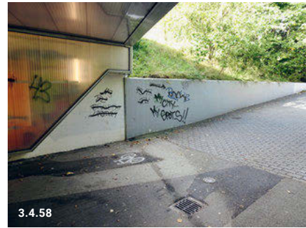
3.4.57 Krogrunden as built 3.4.58 Sharp edge of the singular pavement
