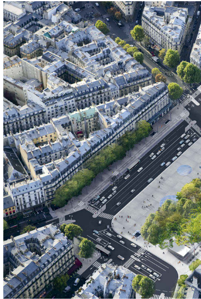
3.1.34–3.1.35 General plan and aerial view of the winning project. TVK et al. , competition entry, November 2009 3.1.36 Pedestrian areas doubled by the project. TVK et al. , diagram, n.d. 3.1.37 From fragmentation to unity of space. Representation of the levels of the square before and after the intervention. TVK and Atec, diagram, n.d.
