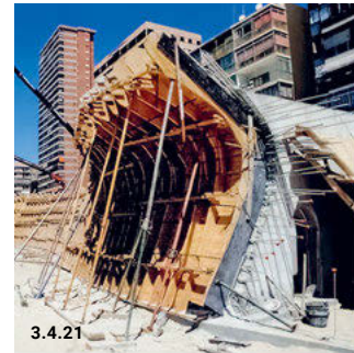
3.4.20 The grid as a design tool materialized in the completed project 3.4.21 Artisanal formwork planted on the ground 3.4.22 Typical segment of the "matrix" 3.4.23 The serial principle applied to the whole length of the promenade 3.4.24–3.4.25 Repetition of a matrix, two similar staircases at two different places on the promenade 3.4.26 Rules and constraints – breakdown of vertical distribution. R: ramp, E: staircase, in bold: existing wall sections preserved
