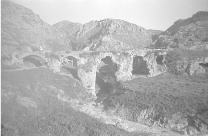
Fig. 3: A bridge of the Trajan-Hadrian aqueduct crossing the Phyrminos Valley (D-DAI-IST-KB 12.696, A. Eckstein).
