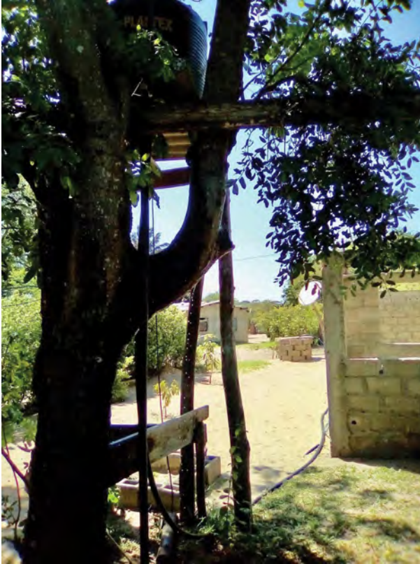
Fig. 4: Infrastructure system of a private water supplier in the district of KaNyaka, Maputo: A borehole in the background feeds water via rubber hoses into a water storage tank from which a further redistribution of the water to different households takes place. (S. Thomschke [2019]).
