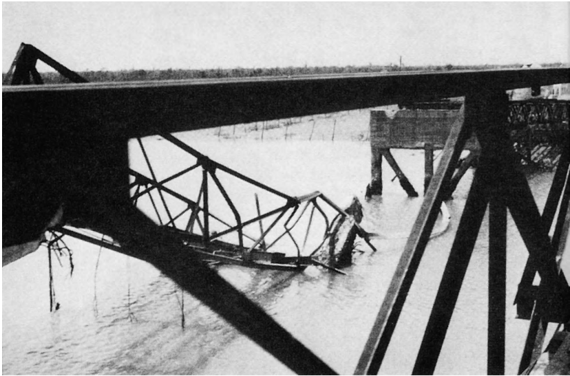
A bridge on Route 15 between Ba Ria and Vung Tau destroyed before our arrival by the Viet Cong.
