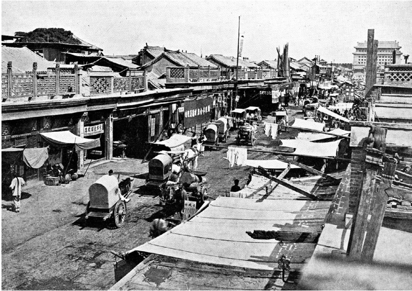
Figure 7.2. Qian Gate Street in the 1900s. Photograph by Sanshichiro Yamamoto. In Peking (Beijing: Yamamoto photography studio, 1906), fig 1.
