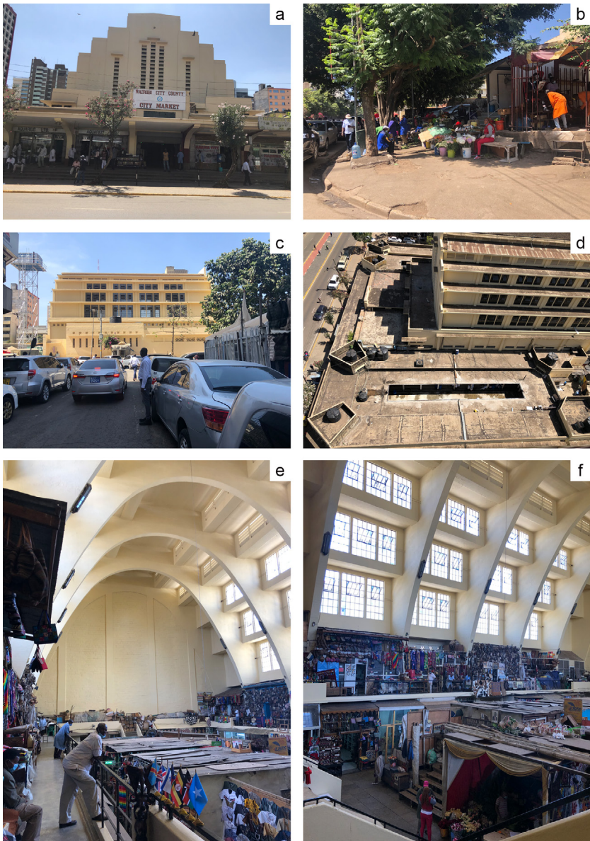
Figure 5.2. City Market from different vantage points. (a): view from Muindi Mbingu Street; (b): view from Koinange Street; (c): view from Market Road; (d): Aerial view from Tubman Road; (e, f): internal views of the market hall. Photographs by author, 2020.
