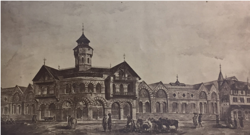
Figure 3.9. The New General Markets in Course of Erection on the Esplanade, 1866. Watercolor by William Emerson. Reprinted (from the original, now lost) in Arthur Crawford, Annual Report of the Municipal Engineer of Bombay for the Year 1867. © The British Library Board, IOR/V/24/2722.
