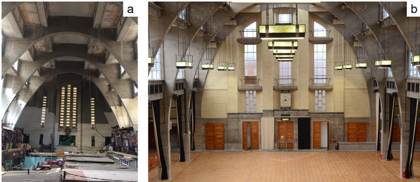
Figure 5.4. Comparison of City Market, Nairobi and Lawrence Hall, London. Note the close similarities between the parabolic arches and stepped fenestration of the two buildings. (a): Photograph of City Market by Samantha Martin, 2019. (b): Photograph of Lawrence Hall reproduced by kind assistance of the Governing Body of Westminster School.
