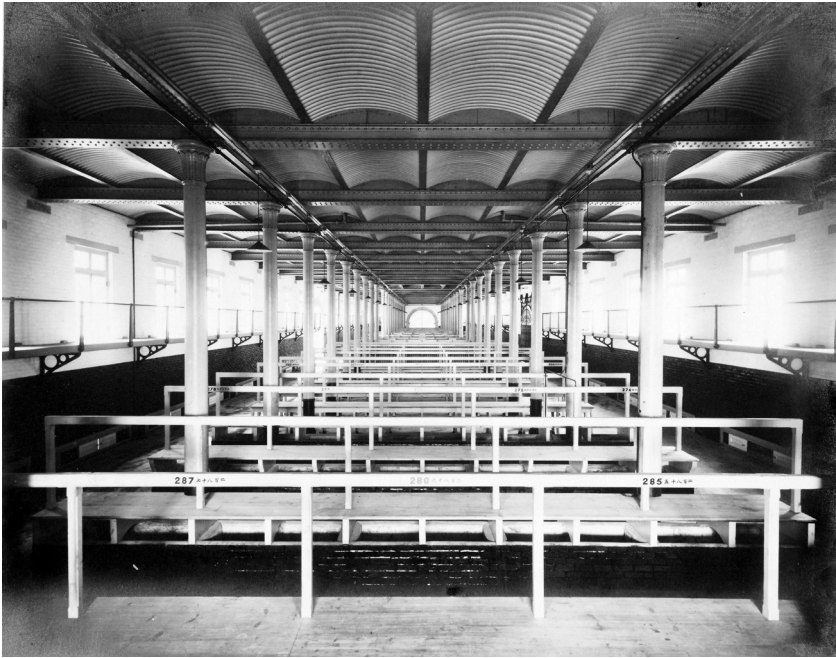
Figure 4.5. Central Market, Hong Kong, 1895. This photograph shows the ground floor of the northern block containing 150 stalls. The vegetable stalls were fitted with tiers of receding shelves, the pork stalls with iron rails and hooks, and some fish stalls with water tanks. Courtesy of the National Archives, London, CO 1069/446 (27).
