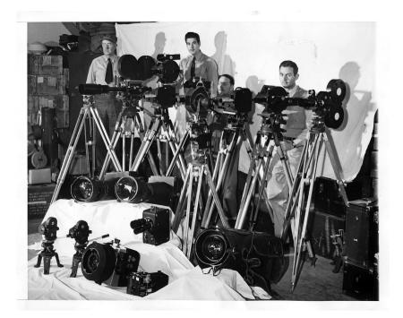
*Figure 2.3* Still and motion picture cameras used during early nuclear testing at the Bikini Atoll. Source: US National Archive and Records Administration.
