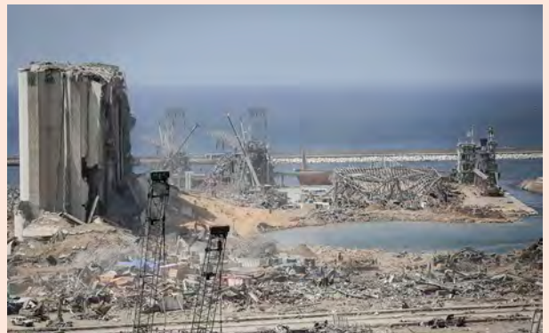
Damage after the Beirut explosion (Wikimedia Commons, photo by Mehr News Agency, CC BY 4.0).
