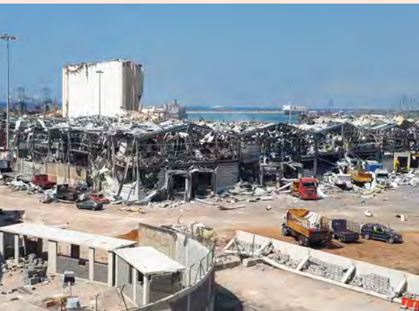
The aftermath of the 2020 Beirut explosions (Wikimedia Commons, photo by Freimut Bahlo, CC BY-SA 4.0).
