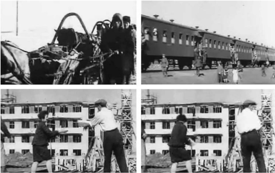
Figure 8.20. Construction newsreels from the Kharkiv Tractor Factory sotsgorod site, 1930. Materials brought to the site by horse cart (top left), worker “volunteers” arrive by train from the city (top right), worker “volunteers” sling bricks (bottom). TsDKFFA Ukrainy, od. obl. 1429, 1447, 1469, 1483, 1486, 1516, 1517, 1529.
