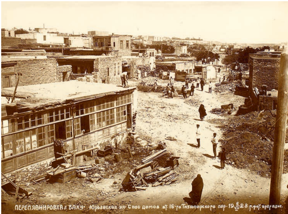
ПЕРЕПЛАНИРОВКА Г. БАКУ. Юрьевская ул. Снос домов от 16-го Тизанинского пер. 19 5 28 ул. Брегдзе. Plate 10. Replanning the City of Baku photo series, documenting the removal of houses along Iur'evskaia Street on July 5, 1928. The elevated vantage point captures the Nagorno Plateau's character before the street was "punched through." Photo: L. Bregadze. RGALI, f. 2991, o. 1, d. 17, l. 125.
