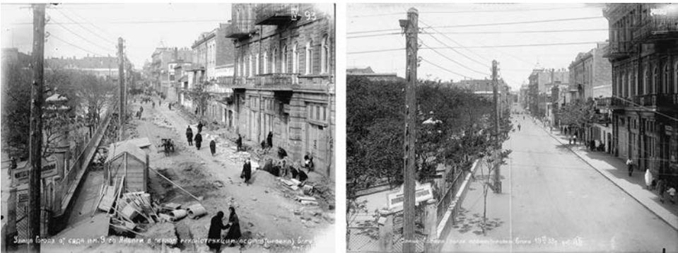
Figure 3.21. Gogol Street during reconstruction (left; February 20, 1933) and after reconstruction (right; May 15, 1933). Photos: L. Bregadze. ARDKFSA, Inv. 5-270, 5-349.
