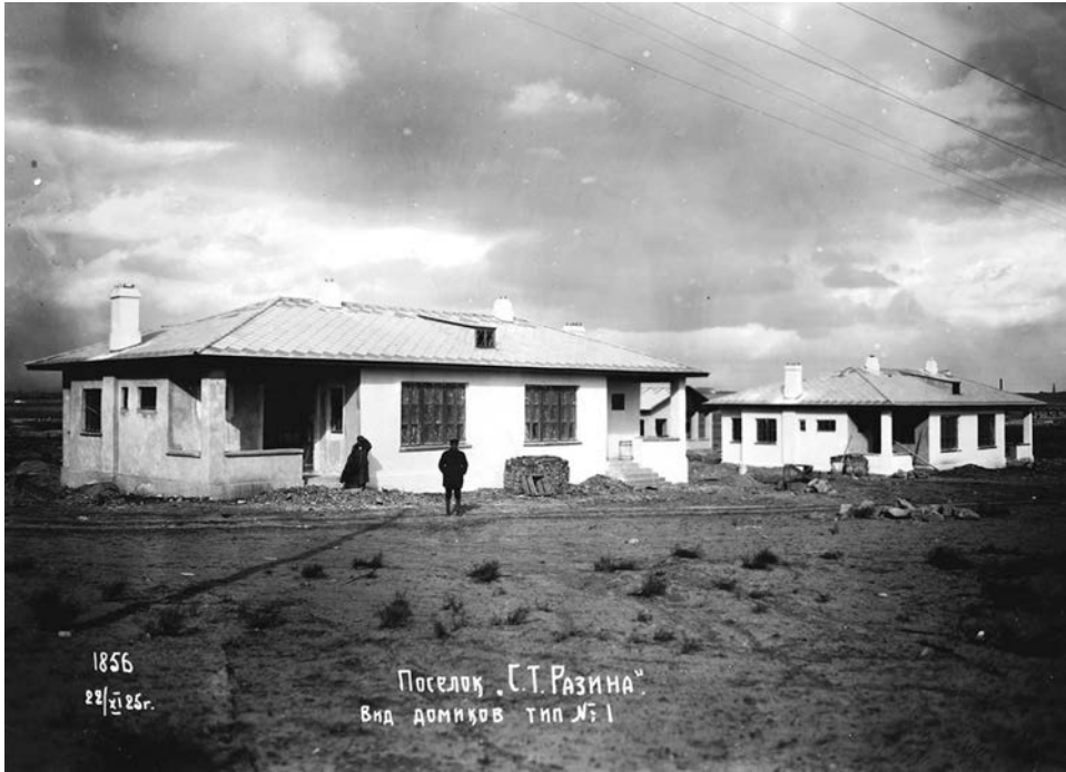
Figure 2.10. Type I houses under construction, Azneft Stepan Razin settlement, Baku, Azerbaijan, November 22, 1925. Architects: Aleksandr Ivanitskii, Viktor Vesnin, Leonid Vesnin, et al. Canadian Centre for Architecture, PH1998:0011:014. Gift of Howard Schickler and David Lafaille.
