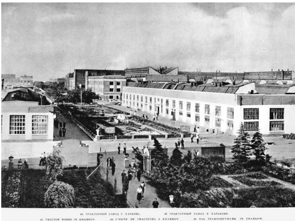
Figure 7.9. West entrance, with the forge shop's butterfly trusses visible in the background, Kharkiv Tractor Factory, Kharkiv, Ukraine, 1930s. Akademiaiia budivnytstva i arkhitektury URSR, Ukraina: Arkhitektura mist i sil (Kyiv: Derzh. vyd. lit. z bud. i arkh., 1959).
