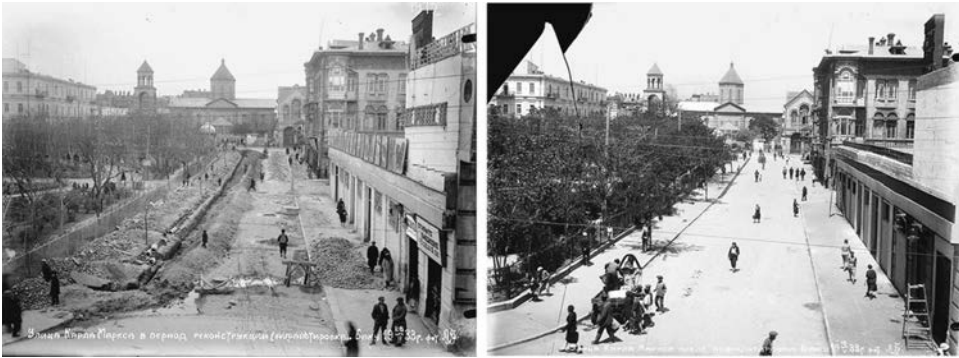
Figure 3.20. Karl Marx Street during reconstruction (left; February 20, 1933) and after reconstruction (right; May 15, 1933). Photos: L. Bregadze. ARDKFSA, Inv. 5-224, 5-223.
