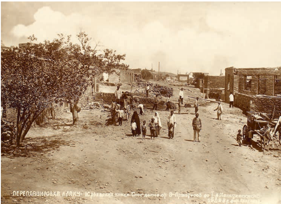
ПЕРЕПЛАНИРОВКА Г. БАКУ. Юрьевская ул. Снос домов от 8-й Пржевальской до 1-й Кавказской ул. 19 5 28 ул. Брегдзе. Plate 11. Replanning the City of Baku photo series, documenting the removal of houses along Iur'evskaia Street on July 5, 1928. The photographer often posed his human subjects to mark the scale of intervention. Photo: L. Bregadze. RGALI, f. 2991, o. 1, d. 17, l. 123.
