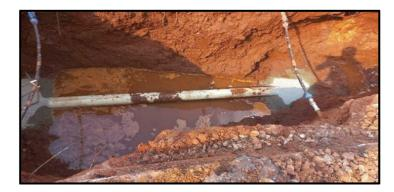
Figure 4. Broken water pipe. source, author's (2022).
