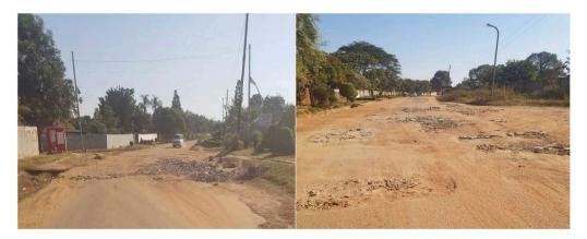
Figure 1. Concrete block debris used to fill potholes on Zambezi Road, Riverside, Kitwe. Source: Authors
