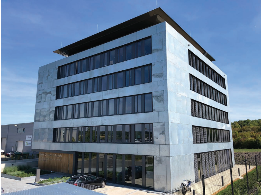
Figure 11.57 Perspective view of Luxembourg building, Christian Bauer & Associés Architects.
