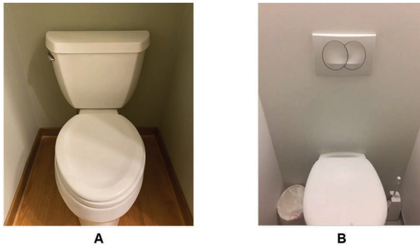
Figure 9.16 Toilets are high-interaction, low-performance impact human-building interactions. (a) Single-flush interface. (b) Dual flush interface (increases user cognitive burden, compared to single flush).
