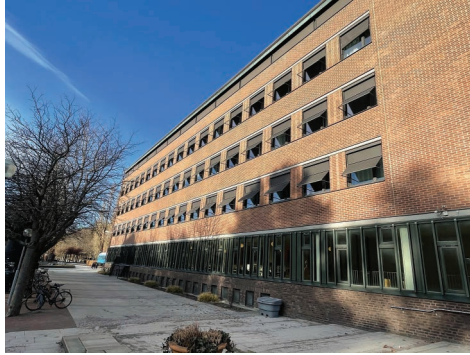
Figure 11.73 Photo of the A-building exterior space.
