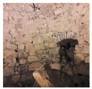
Figure 6 – Underground room at *limonaia* Fondo Campagnola (Gargnano) to collect and drain the water springing from the rocks.
