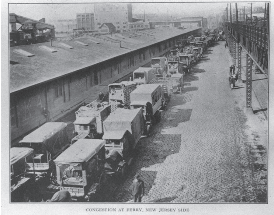
Fig. 4.1. Trucks lined up for the ferry in Hoboken (c. 1918–1919). ( Photograph reprinted by permission of the Hoboken Historical Museum. )
