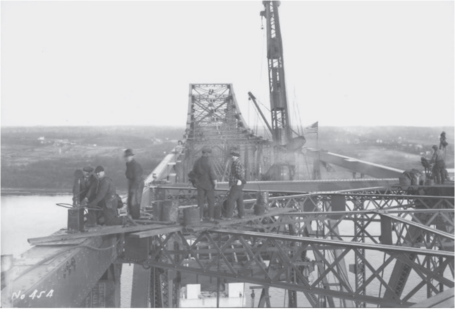
Fig. 7.1. Construction of the Outerbridge Crossing.
