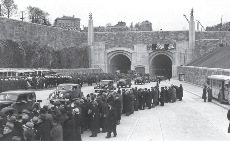
Fig. 2.8. The second tube of the Lincoln Tunnel opened in 1945. (Photograph reprinted by permission of Port Authority of New York and New Jersey.)
