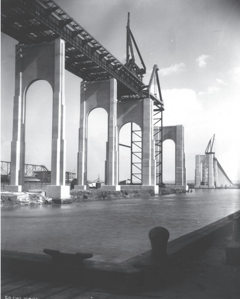
Fig. 7.2. Goethals Bridge construction.
