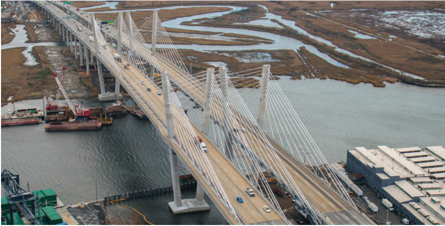
Fig. 7.6. The two spans of the new Goethals Bridge opened between 2017 and 2018. (Photograph reprinted by permission of Port Authority of New York and New Jersey.)
