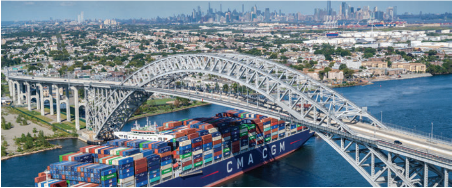
Fig. 7.9. One of the world's largest container ships sailed under the Bayonne Bridge in 2020.
