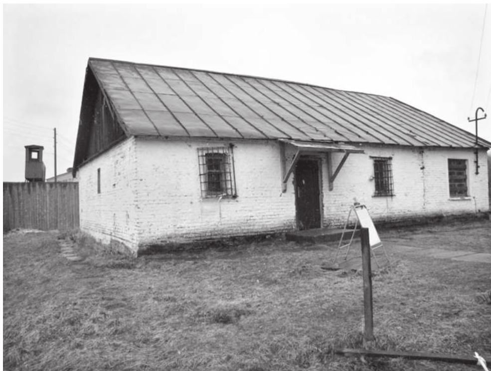
Figure I1.3. ShIZO (penal isolation building) in the Kuchino concentration camp where I stayed for the quarantine (contemporary view). Photo credit: Iliia Buianovsky.
