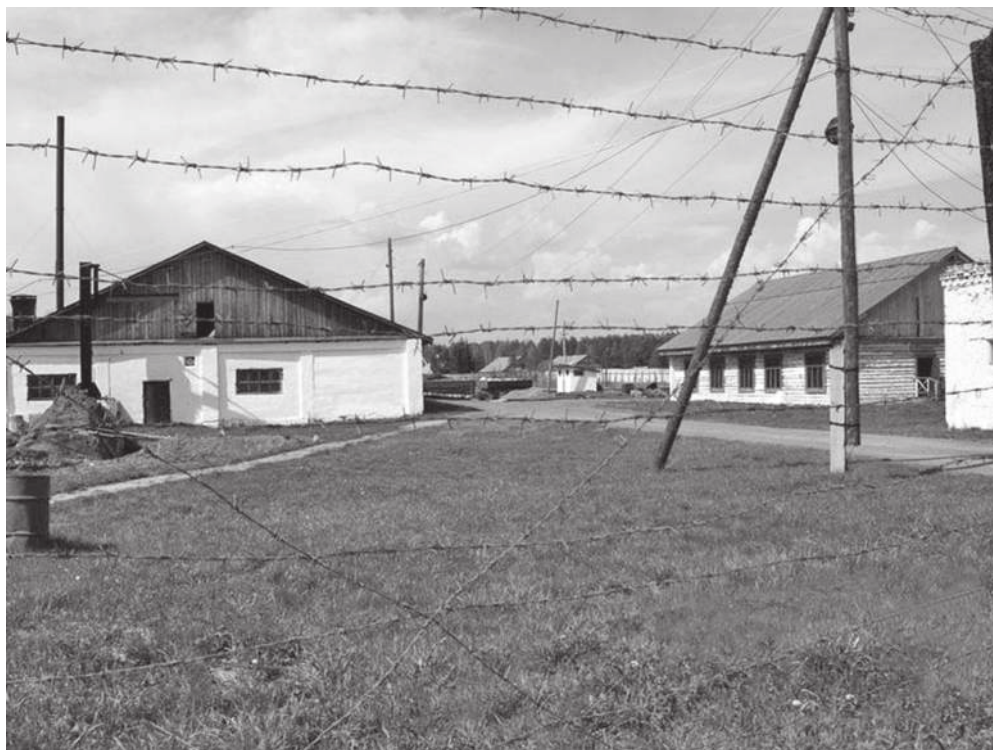
Figure 6.2. The work zone.
